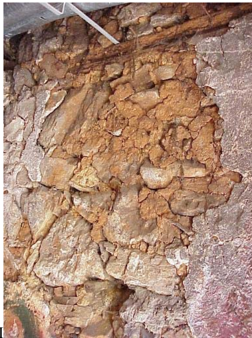
Figure 5 – Typical examples of masonry for external walls
