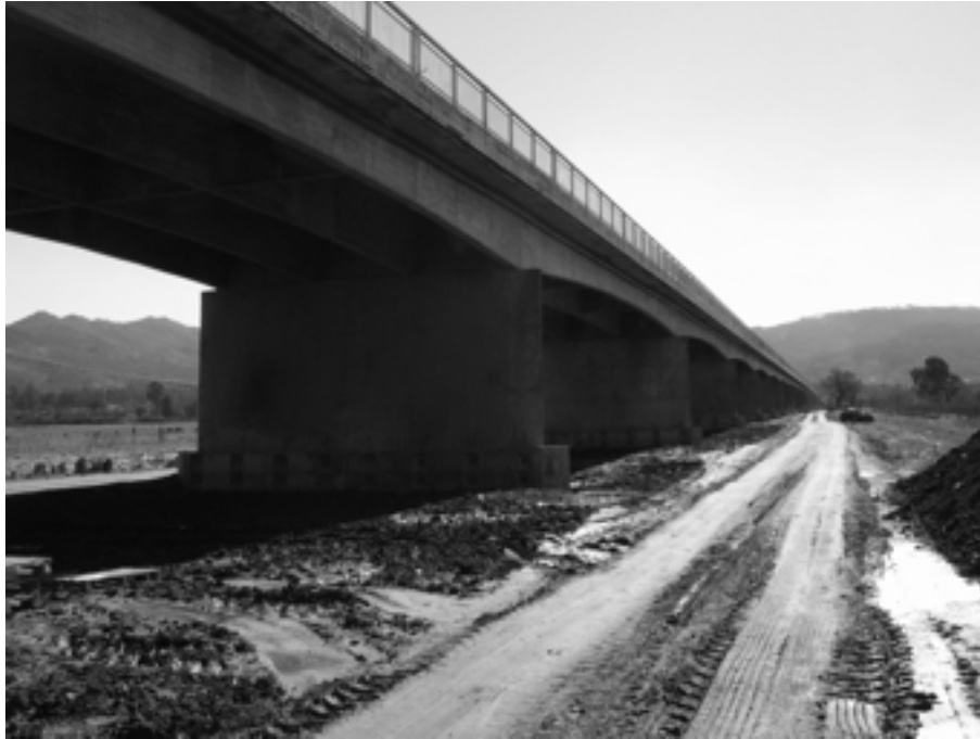
Figure 5.1 – Overview of the Lanheses Bridge.
