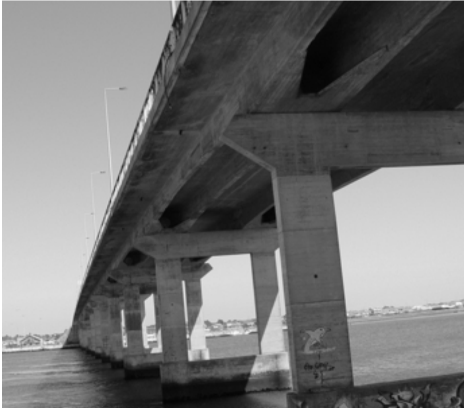
Figure 5.2 – Overview of the Barra Bridge.
