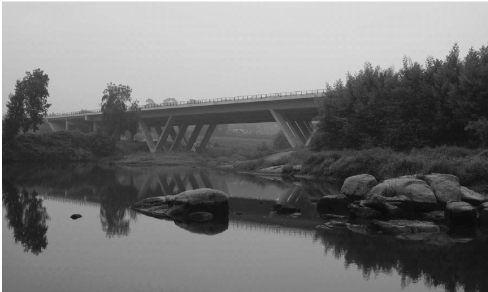
Figure 5.3 Overview of the Bridge over Ave River.
