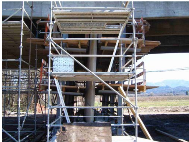
Figure 6.1 - Example of scaffolding system used to access the test site
