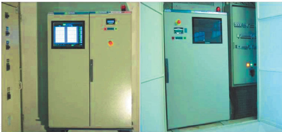
Figure 16. Two of the four final prototypes of Shunt Active Power Filters.
