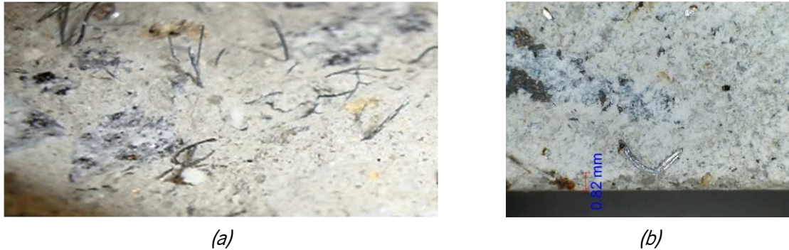
Figure 6.15 – Crack surface of specimens after 3 months of chloride immersion (Series V): (a) General aspect of RSF (b) Corrosion sign on RSF near the exposed surface
