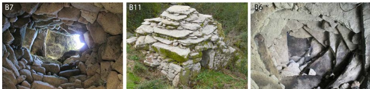
Figure 1: Examples of the study area’s corbelled domes. Examples from branda of Gêmea Group B’s buildings.
