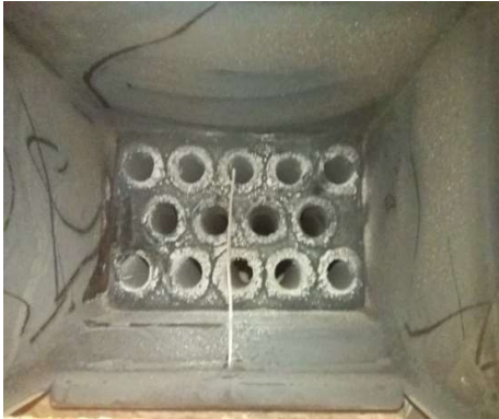
Figure 3.2. Heat exchanger pipes, bottom view.
