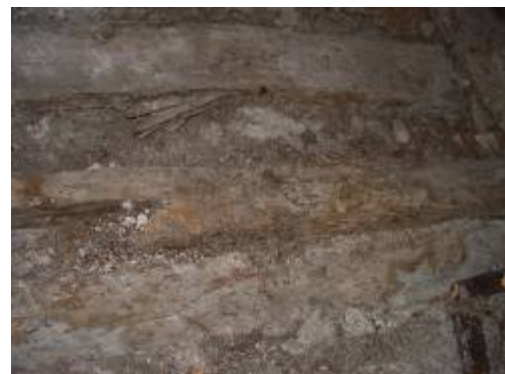
Fig. 3: Details of the generalized infestation and the irregularity of the cross section of the ribs due the attack
