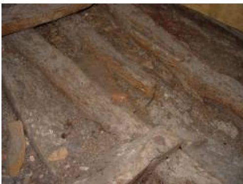
Fig. 3: Details of the generalized infestation and the irregularity of the cross section of the ribs due the attack
