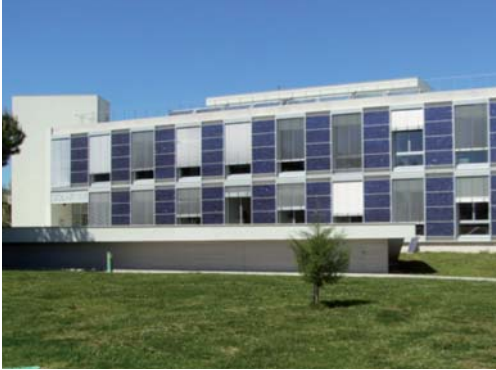
Solar XXI Building in Lisbon generates 80% of its energy consumption. Innovative energy concepts also take place in the surroundings. Source: "INEGI 2009" – Portugal
