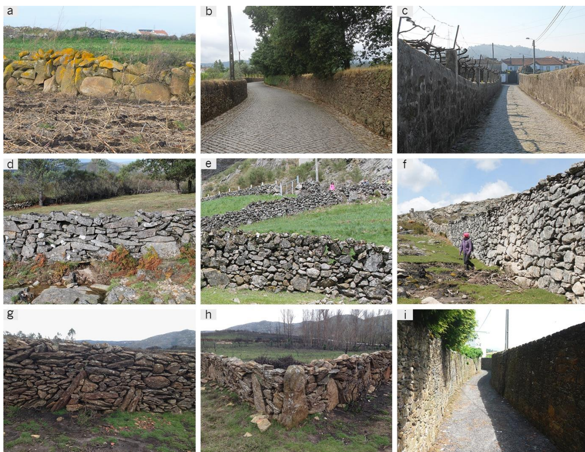
Fig. 5.20 - Images of different farm walls seen during the exploratory visits. In the lowland: (a) low boundary farm wall in granite (Póvoa de Varzim); (b) medium-height boundary (on the right) and high full protection farm wall in granite (on the left) (Barcelos); (c) high full protection farm wall in granite (Barcelos); (i) full protection high farm wall in schist (Barcelos). In the highlands: (d) low animal intrusion protection farm wall in granite (Peneda mountain range, Arcos de Valdevez); (e) medium-height boundary and animal intrusion protection farm wall in granite; (f) wolf pit trap high farm wall in granite (Peneda mountain range, Arcos de Valdevez); g and (h) low animal intrusion protection farm walls in schist (Agra mountain range, Viana do Castelo).
