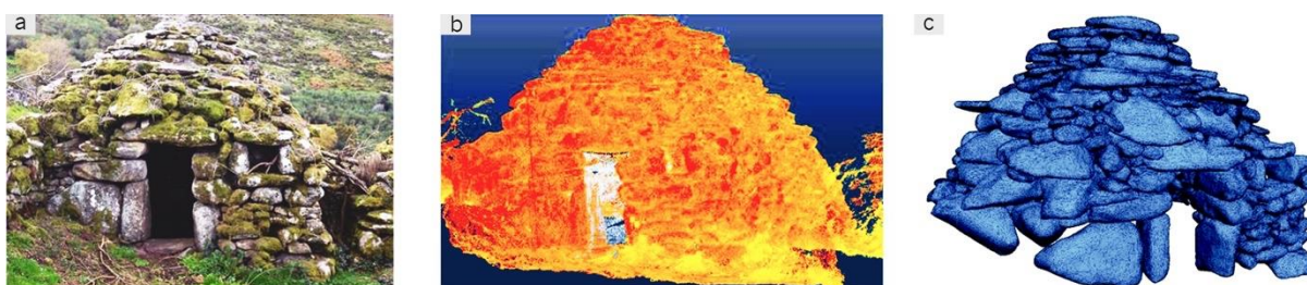
Fig. 9.27 – Sequence of task for the safety analysis: (a) inspection and dynamic identification of case study under analysis for structural safety; (b) point cloud created by laser scanning (author Dr. Belén Riveiro); (c) mathematical model based on the point cloud (author Dr. Belén Riveiro).
