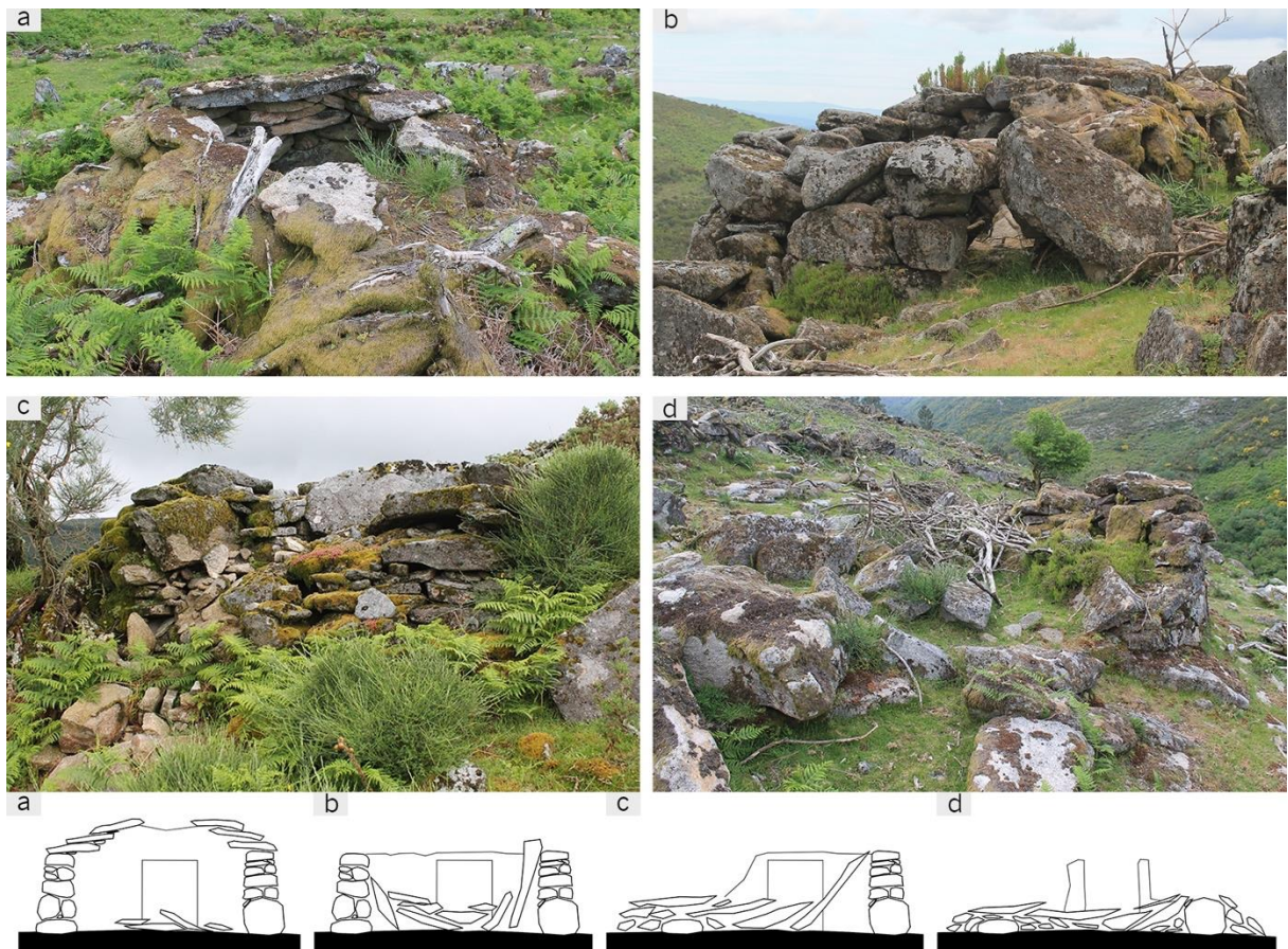
Fig. 9.35 - Examples of ruined small-size livestock shelters ( “branda” of Rio Covo, Sistelo): (a) domes' partial collapse due to masonry unit's rupture; (b) building's corbelled dome in complete ruin (collapsed inward), but showing masonry walls in good condition; (c) masonry walls' partial collapse due to dome's inwards collapse; (d) building in complete ruin (partial reuse of stone).
