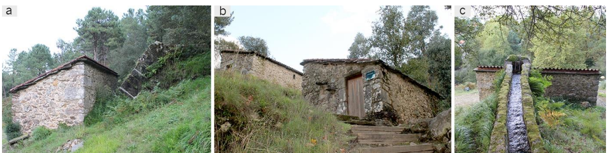
Fig. 5.16 – Example of mountain watermill rehabilitated for museum, feed by conducted water system: (a) masonry pipe named “ cubo ”, that feeds the horizontal wheel; (b) view of the mills aligned down slope to maximize water strength and management; (c) water aqueduct, named “ levada ”, that feeds the masonry pipe.
