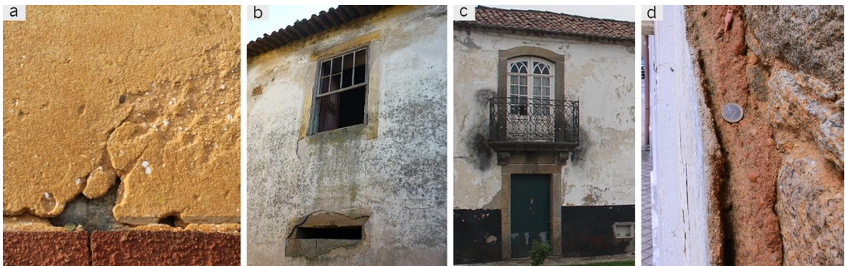
Fig. 6.11 – Examples of renders and painting: (a) “ saibro ” yellowish and reddish render (Laúndos, Póvoa de Varzim); (b) white lime painted renders with painted yellowish frames and bands (Balazar, Póvoa de Varzim); (c) façade showing a lower darker band (Barqueiros, Barcelos); (d) example of a thick render with inner layers in “ saibro ” render, and an external layer of lime render (Barcelos).
