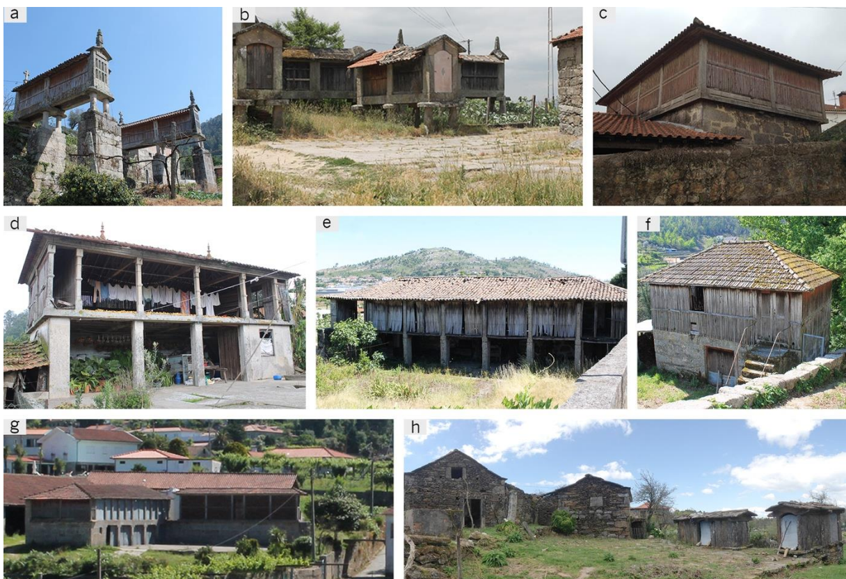
Fig. 5.9 - Examples of grain production infrastructures seen during the exploratory visits: (a) two “ espigueiros ” placed over the road and facing a threshing floor (Paço Vedro de Magalhães, Ponte da Barca); (b) group of “ espigueiros ” placed around a common highland threshing floor (Ermida, Ponte da Barca); (c) “ sequeiro ” (Vilar de Figos, Barcelos); (d) “ sequeiro ”, with built in “ espigueiros ” on both sides, and threshing floor located outside the farmstead (Paradela, Barcelos); (e) large-size “ sequeiro ” and threshing floor (Sequeira, Braga); (f) isolated “ sequeiro ” with threshing floor (Vila Nova de Muía, Ponte da Barca); (g) isolated grain production compound formed by a large a “ sequeiro ” with built in lateral “ espigueiros ”, a large-size “ espigueiro ” and threshing floor (Rio Covo de Santa Eulália, Barcelos); (h) group formed by threshing floor, threshing floor house and “ espigueiros ” (Arga de Cima, Caminha).
