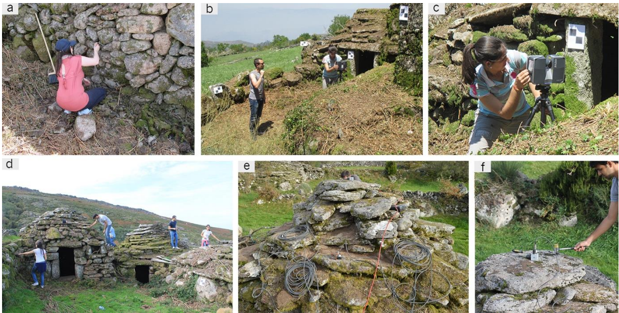
Fig. 9.24 – (a), (b) and (c) images from the laser scanning survey; (d) visual inspection and preparation for a laser scanning and dynamic identification surveys; (e) and (f) images from the dynamic identification survey.
