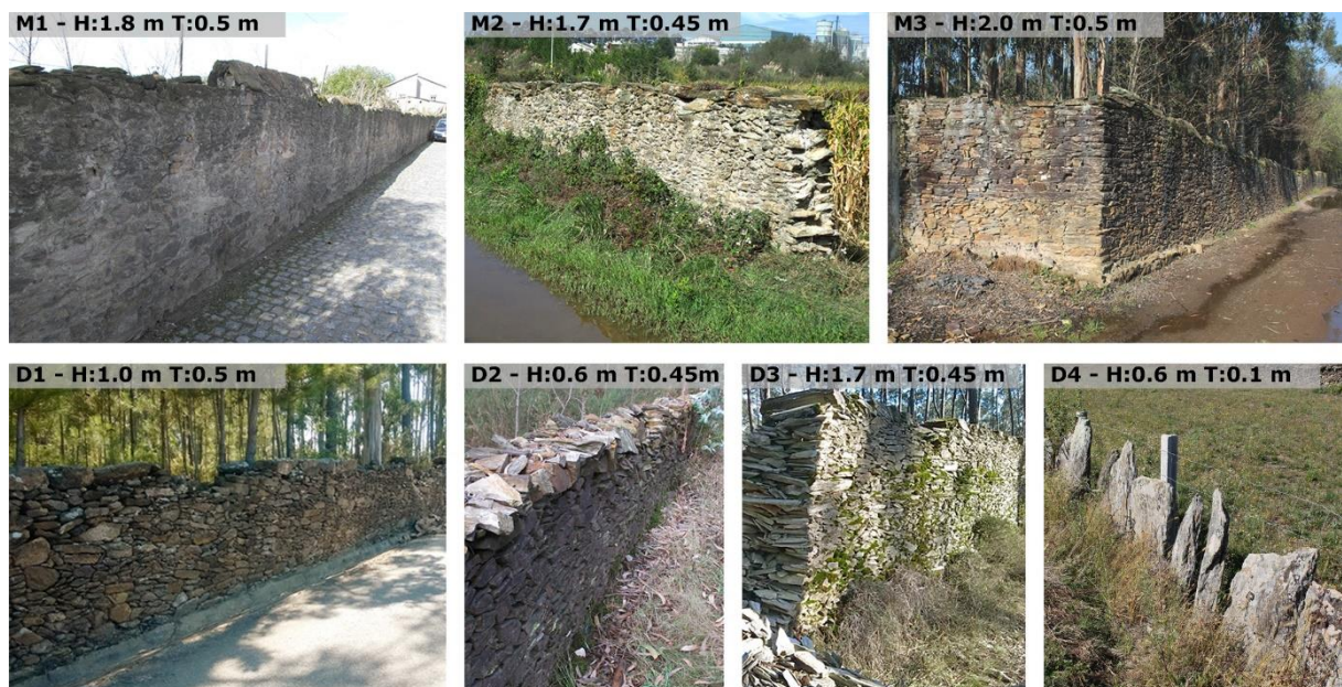
Fig. 9.5 – Examples of farm walls with mortar (group M) and dry joints (group D). Average height (H) and thickness (T) dimensions are presented in each image.
