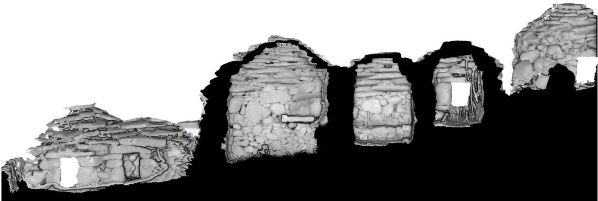
Fig. 9.37 – Laser scanner generated cross-section, showing deformed masonry walls due to overlapping corbelled domes (from left to right).
