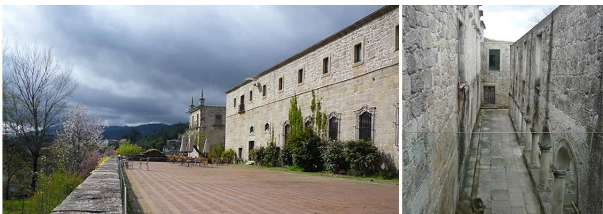
Fig. 2.10 – Transformation of the St. Mary of Bouro monastery into an hotel, by rehabilitating and modernizing specific areas of the building, and keeping others as stabilized ruins not to alter the present aesthetics (Terras de Bouro, Portugal).
