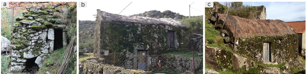
Fig. 5.27 – (a) example of corbelled dome watermill (Padrão, Arcos de Valdevez); b and (c) examples of “ branda ” houses still with original straw roofing (“ branda ” of Busgalinhas, Gavieira, Arcos de Valdevez).
