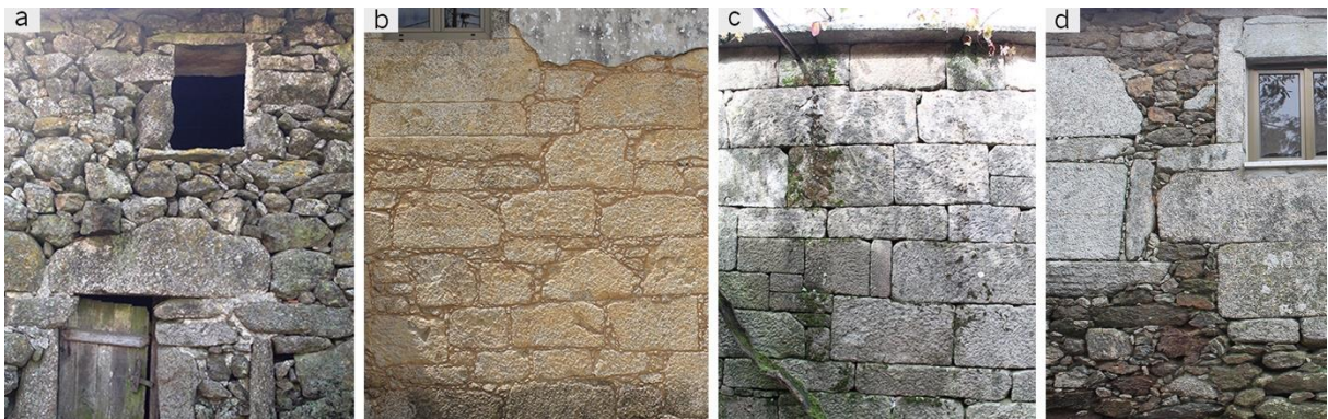
Fig. 6.7 – Different types of superficial masonry textures observed during the exploratory visits: (a) random joints (rubble masonry); (b) uncoursed joints (irregular shaped stone blocks); (c) coursed joints (ashlars or large regular stone blocks); (d) mixed joints (combining different types of schist and granite stone blocks).
