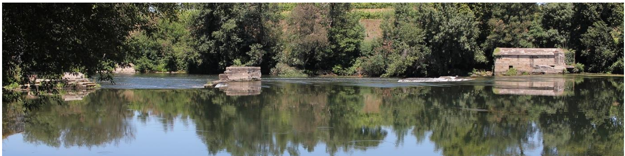
Fig. 5.15 - Example of a ruined watermill group built in the Cávado river on top of the small dam wall. These were mills of vertical wheel, with “ quebra-mar ” reinforcements. The image shows the two remaining mills (left and right), and the foundations of other two (centre).
