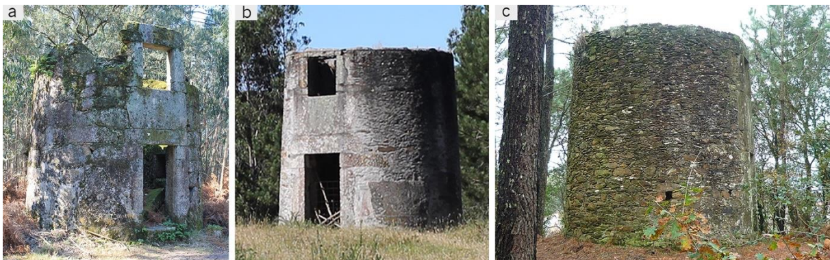
Fig. 5.18 - Examples of windmills in ruins seen during the exploratory visits: a and b - granite constructed mills (Monte of Fralães and Cristelo, Barcelos); (c) schist constructed mills (Barqueiros, Barcelos).
