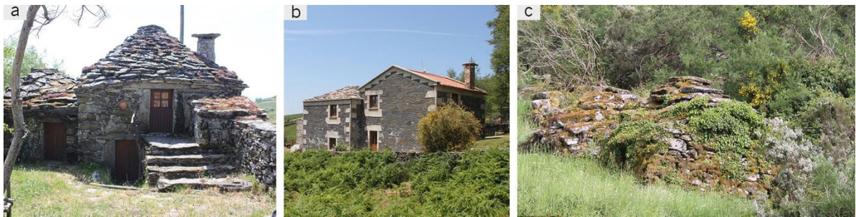
Fig. 9.41 – Examples of human caused damage: (a) and (b) severe and full loss of authenticity of both buildings and site caused by poor interventions (“branda” of Santo António of Vale de Poldros, Monção); (c) group of corbelled dome buildings discovered in “branda” of Gêmea during the cleaning operation.
