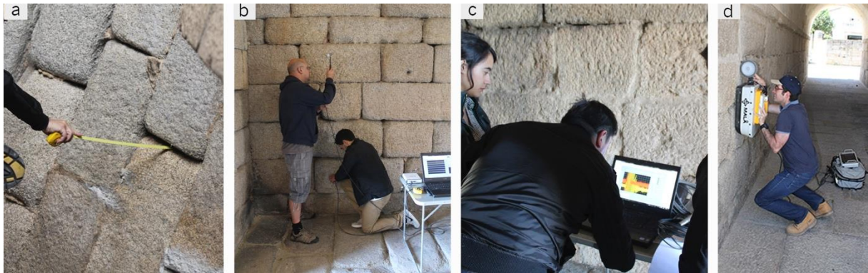
Fig. 2.8 – Examples of different on-site structures analysis techniques, applied to heritage buildings (Almeida city wall, Portugal): a – visual inspection of damage; b and c – dynamic identification through sonic testing; d – inspection by geo-radar [50].
