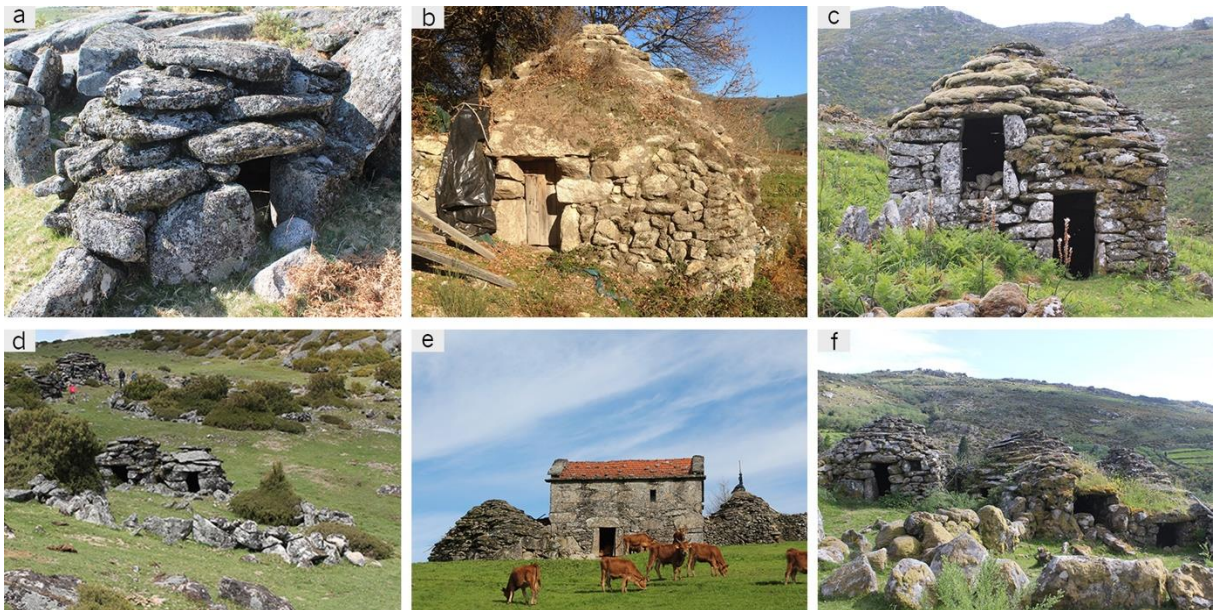
Fig. 5.26 – Examples of corbelled dome isolated and grouped buildings (see Fig. 5.25): (a) small one-storey shelter; (b) larger one-storey shelter with dome covered with earth; (c) two-storey shelter; (d) simple group; (e) composed group; (f) complex group.
