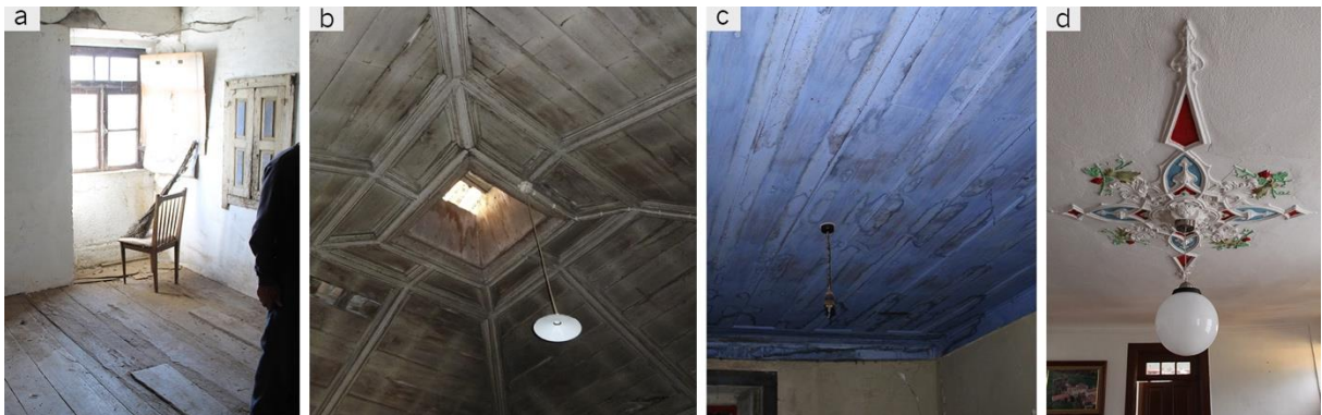
Fig. 6.12 – Detailed view from the interior of visited vernacular buildings: (a) view of a bedroom (Fonte Boa, Esposende); (b) “ masseira ” ceiling without paint (Barqueiros, Barcelos); (c) flat ceiling built in painted timber panels (Barqueiros, Barcelos); (d) plaster “ tabique ” ceiling with a plaster decorative element at the centre (Paradela, Póvoa de Varzim).
