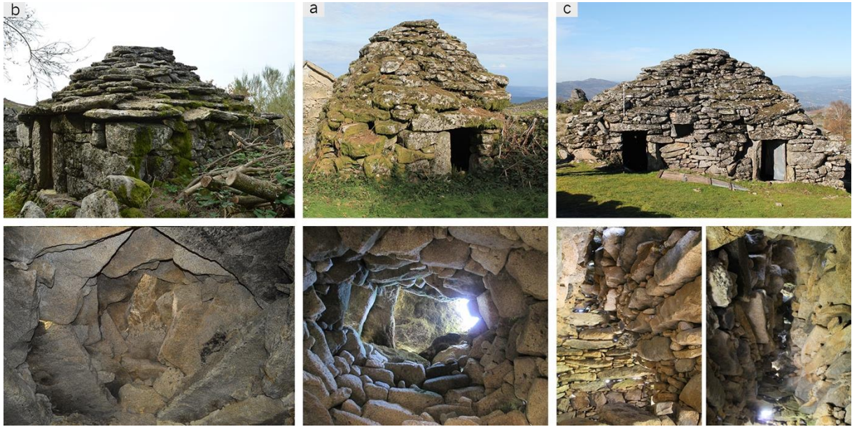
Fig. 9.33 – External (above) and internal (below) view of examples of different corbelled domes identified during the field survey: (a) taller dome built with parallelepiped and irregular shaped stone blocks (“ branda ” of Gêmea); (b) lower dome built with large plate shaped stone blocks (“ branda ” of Gêmea); (c) corbelled vault building with double chamber (“ branda ” of Alhal).
