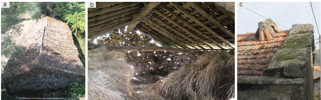
Fig. 6.2 – Images of three gable roofs: (a) external view of a roof with “ lusa ” tiles (Vale, Arcos de Valdevez); (b) internal view of the structure of a gable roof covered with “ lusa ” tiles (Lindoso, Ponte da Barca); (c) detail view of a roof originally covered with straw replaced by “ marselha ” tiles, showing the granite wind protection capstone, and chimney built in “ lusa ” tiles.
