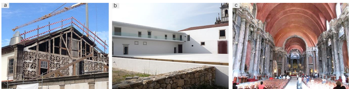
Fig. 2.6 – Examples of different rehabilitation operations: a – adaptation and upgrade of an heritage building (Guimarães, Portugal); b – introduction of a new use and new elements into a ruin area of the Tibães Monastery (Braga, Portugal); c – rehabilitation and reconstruction of the St. Domingos church, keeping the memory of the fire that ruined it (Lisbon, Portugal).
