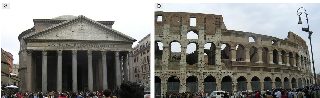
Fig. 2.9 – Monumental heritage preservation examples: a – preservation of the historical damage in the Pantheon (Rome, Italy); b – stabilization and reconstruction intervention using new but clearly distinguishable materials in the Colosseum (Rome, Italy).
