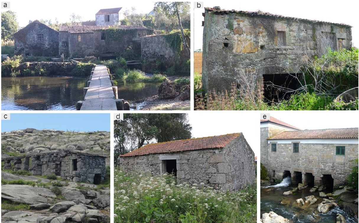
Fig. 5.14 - Examples of watermills observed during the exploratory visits (in ruins or disabled): (a) large milling complex with combined vertical and horizontal wheel systems (Antas, Esposende); (b) schist individual mill of horizontal wheel (Rio Tinto, Barcelos); (c) example of a mountain range “ cubo ” mill of horizontal wheel, belonging to a group of several mills align down slope (Agra mountain range, Caminha); (d) individual mill of several horizontal wheels (Aguçadoura, Póvoa de Varzim); (e) large mill with several horizontal wheels integrated in a farmstead (Medros, Barcelos).
