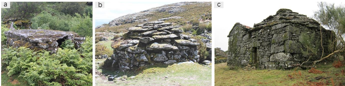
Fig. 5.23 – Examples of different corbelled domes and construction quality of the highland vernacular heritage: (a) poor construction quality; (b) low construction quality; (c) improved construction quality.
