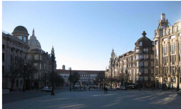
Porto: Aliados Avenue Slope: 9% Normalization: 0.66
