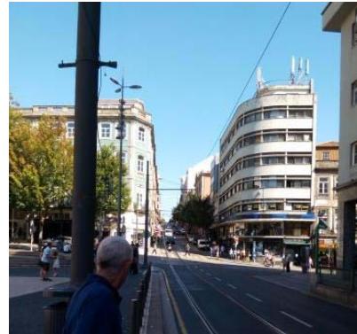
Porto: Passos Manuel Street Urban Space, & Buildings Façade (Two compounds) Normalization: 0.69
