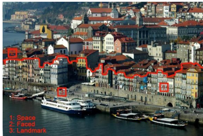
Figure 5-6: Visual Dimension quality of Cais da Estiva street (Porto) using photograph
