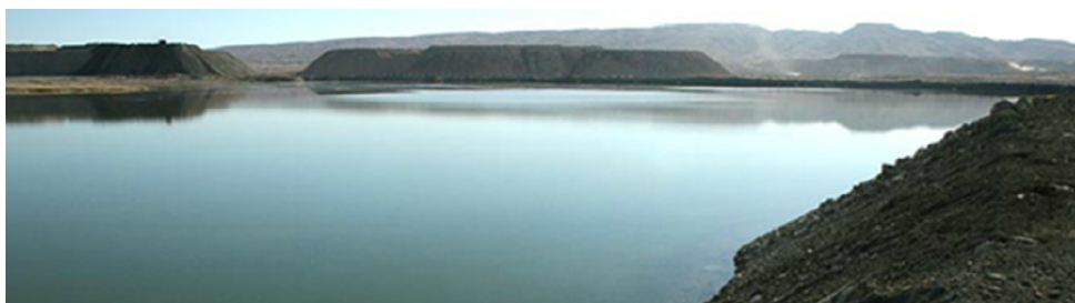
Fig. 1. Tunisian phosphate washing waste pond.
