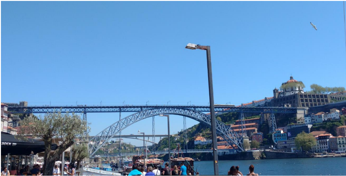
Figure 21 – Luiz I bridge (author, 2017)
