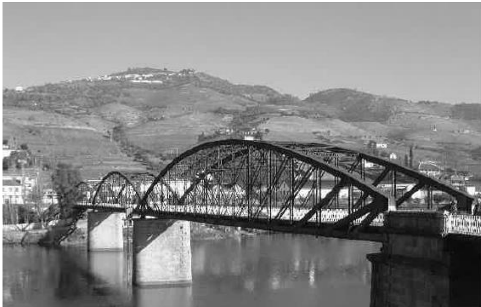
Figure 23 - Pinhão bridge (Correia, 2014)
