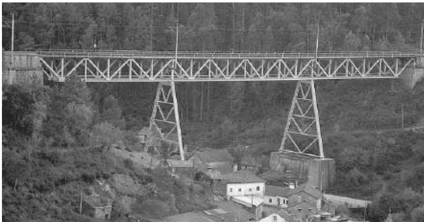
Figure 25 - Trezói railway bridge (Correia, 2014)
