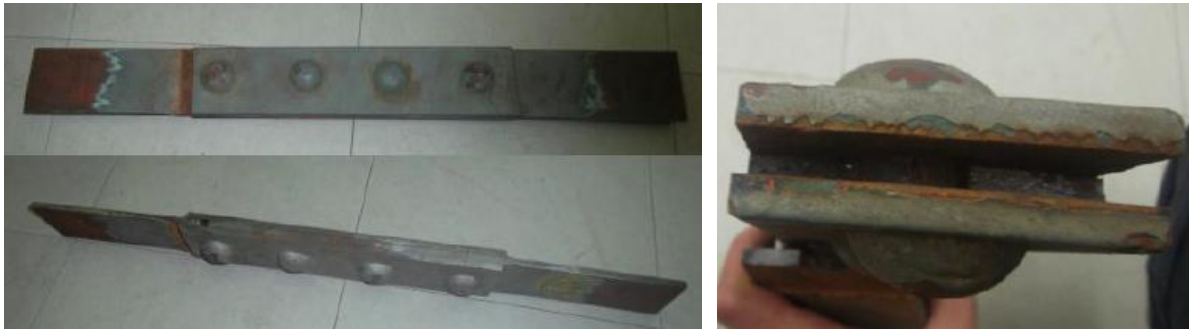
Figure 30 - Photos of the specimens with double shear riveted connections, cut from Viana bridge (Correia, 2014)
