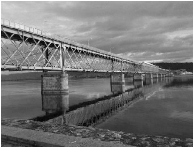
Figure 24 - Viana bridge (Correia, 2014)
