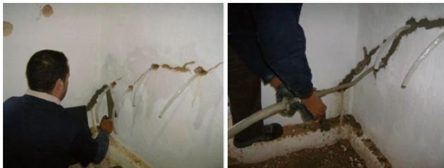
Figure 24- Grout injection used to repair of cracks (Figueiredo et al. , 2013)
