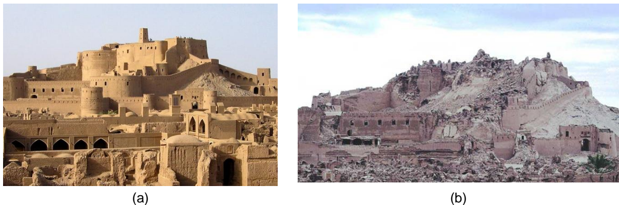
Figure 5- Arg-e-Bam (UNESCO world heritage as the largest adobe site): (a) before and (b) after earthquake in 2003
