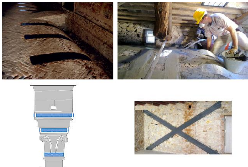
Figure 29- Examples of FRP-composites application on existing buildings (Valluzzi et al. , 2014)
