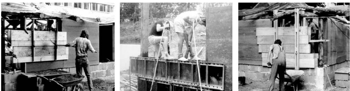
Figure 8- Rammed earth construction process (Minke, 2006)
