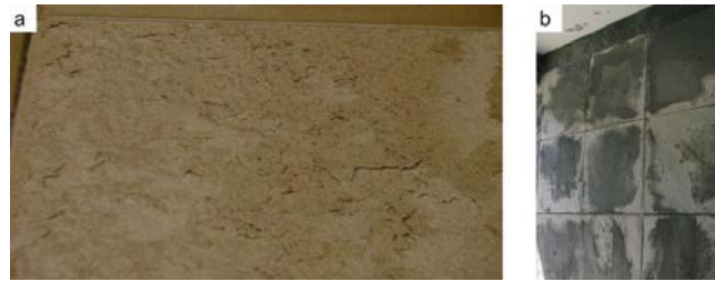
Fig. 2. Erosive features on (a) porous limestones and (b) schist rocks on a porch-like structure (erosion concentrated along joints suggesting solutions circulation).
