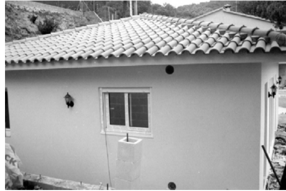
Figure 2. Exterior view of a lightweight exterior wall.
