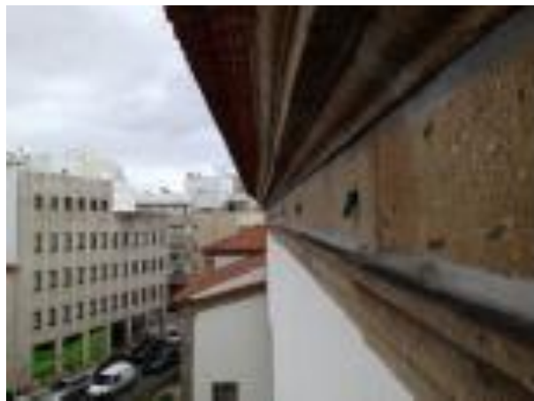
Figure 51 - North wall view from the main façade (Betzer et al., 2014).
