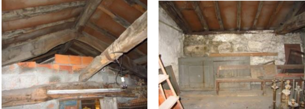
Figure 53 - Roof structure accessible from the north wing area (Betzer et al., 2014).
