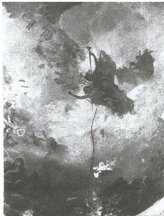
Figure 51 – Cracks in the lateral dome (Schiros, 1975)
