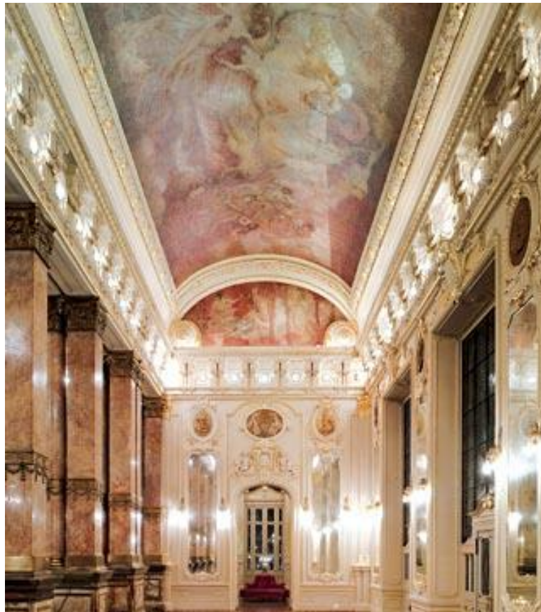
Figure 52 – Barrel vault over the foyer (Eder Santos Carvalho, 2012)
