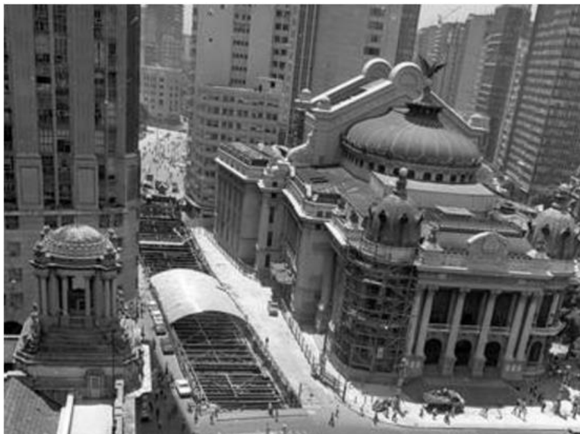
Figure 48 – Construction of the Cinelândia metro station (O Globo, 1996)
