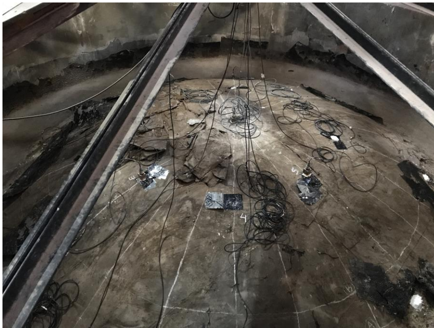
Figure 69 – View of the accelerometers for Setup 1 of the lateral dome
