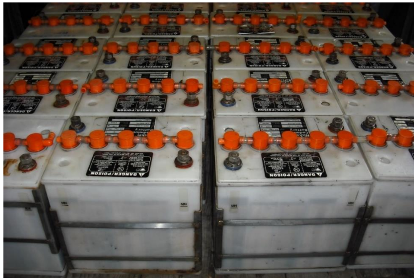
Figura 2.8 - Pack de baterias Ni-Cd [41] (fonte: Electric Vehicles of Washington )
