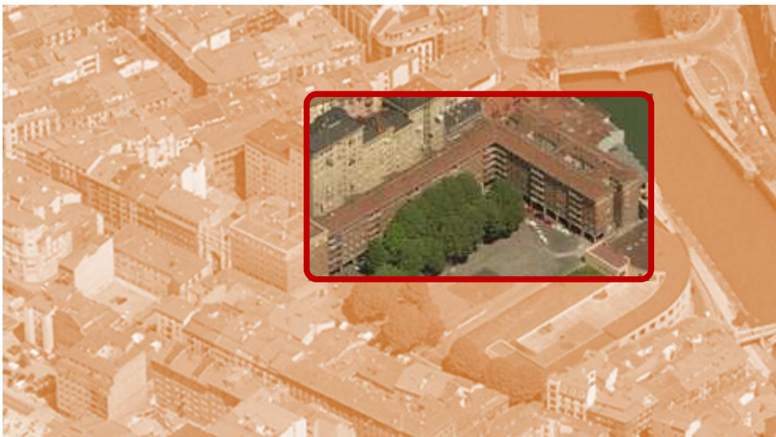
General view of the building
