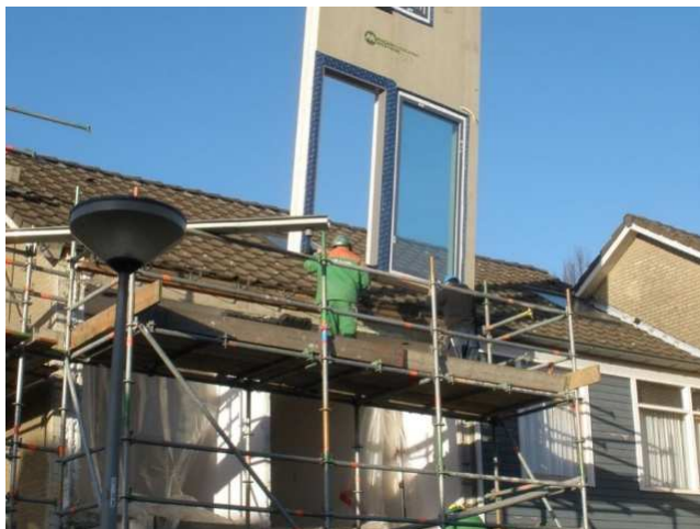
The houses during renovation – facade installation
