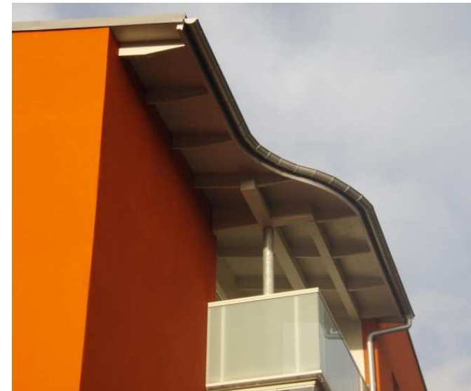
Extended eaves and balcony after renovation
