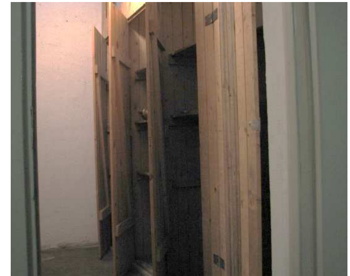
Before renovation – basement storerooms
