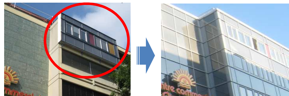
Pre-fabricated solar facade system from gap-solution
