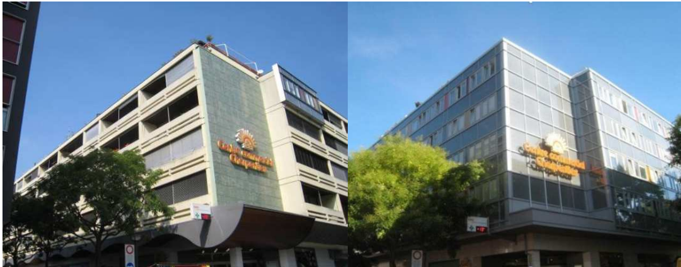
South and East facades - Before renovation
