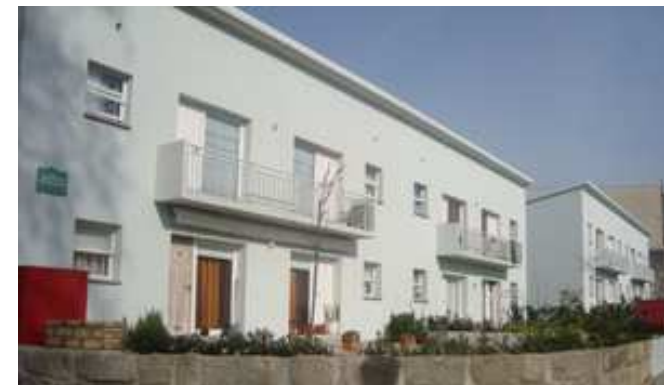
Building after the renovation process
