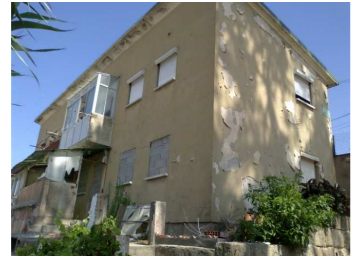
Building before renovation
