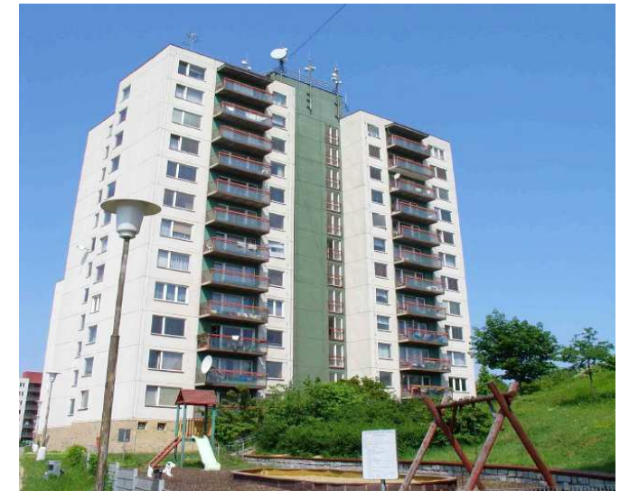
Eastern view of Koniklecová 4 block-of-flats before the renovation. [2]
