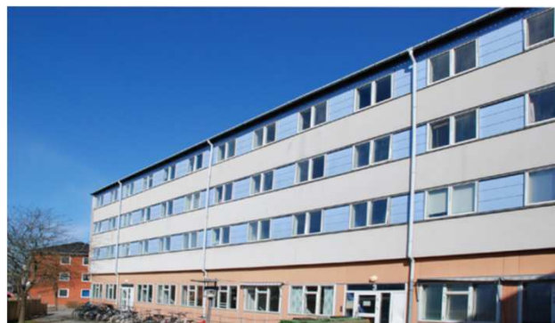
Block A before renovation
