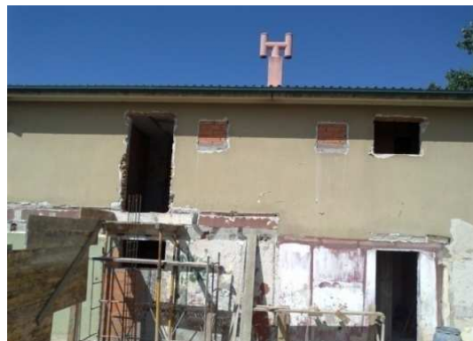
Building during the renovation process
