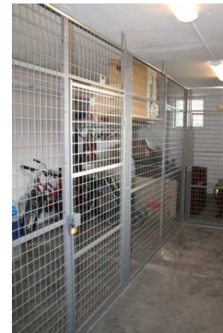
After renovation – basement storerooms
