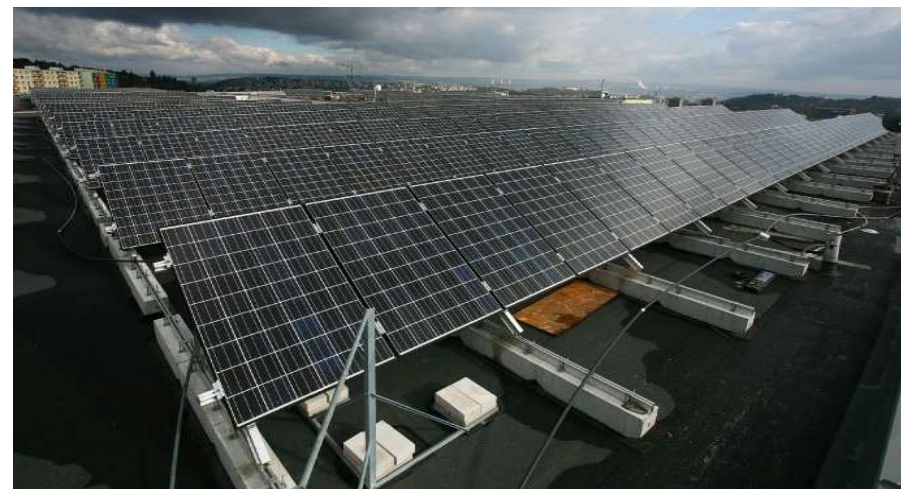
Photovoltaic panels installed on the roof of the A block. [2]
