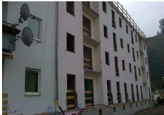
Facade during the renovation
