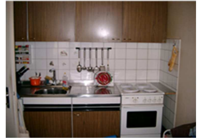
Kitchen before renovation
