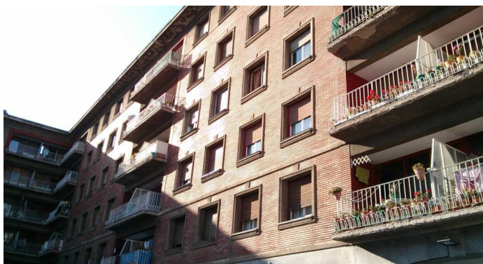
Building façade before renovation
