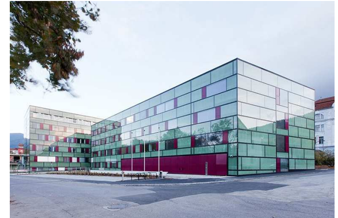
Building after the renovation (© Markus Kaiser, Graz)
