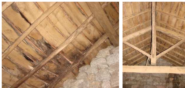
Roof condition and characteristics
