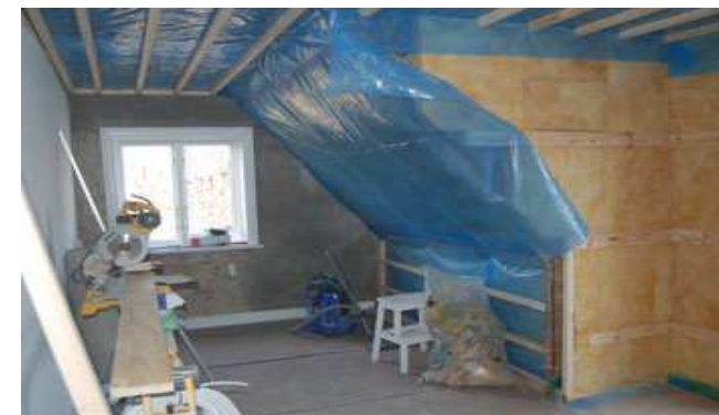
Insulation of mansard walls and lost space walls in attic incl. vapour barrier and internal insulation of the pediment
