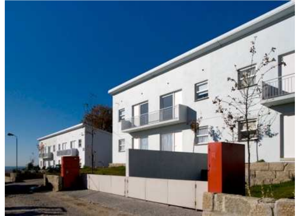
Front facade of the renovated buildings
