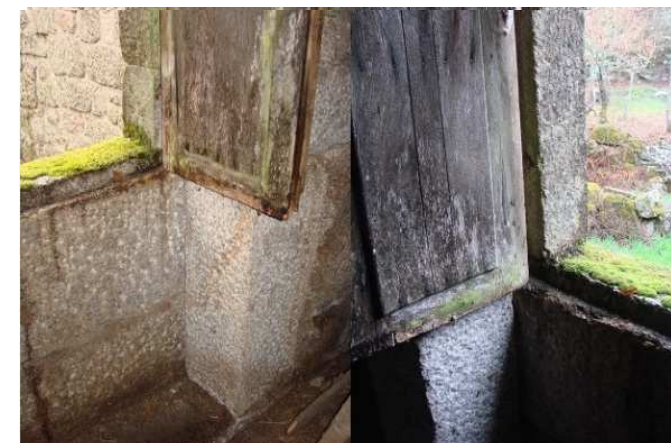
Existing window sills
