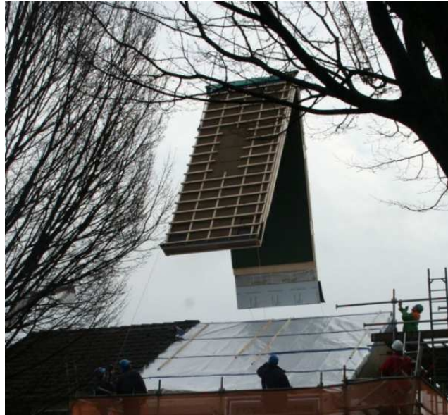
The houses during renovation – roof installation
