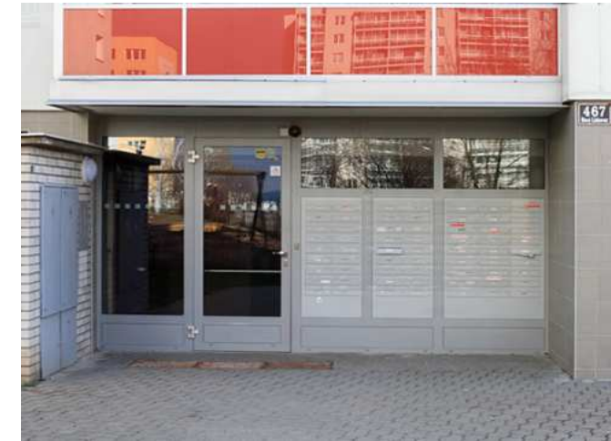
Main entrance before (left) and after (right) renovation. [2]
