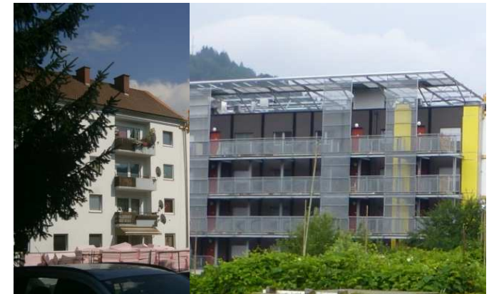
Facade – before and after the renovation
