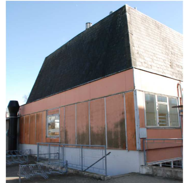
Block B before renovation.
