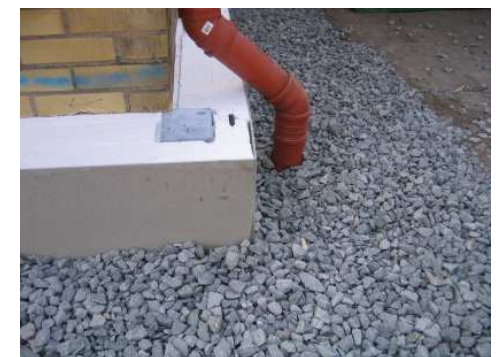
Added insulation to the foundation
