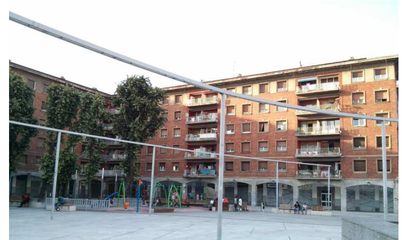
Building before renovation
