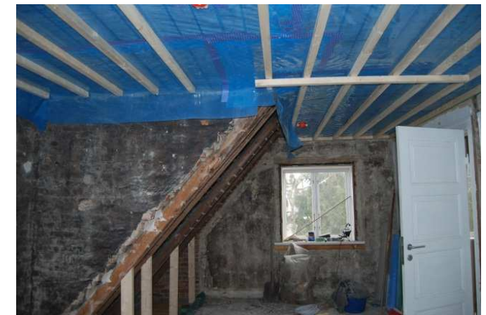
The new vapour barrier on the loft
