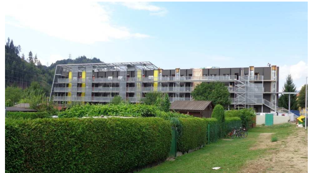
A few days later – building envelope of the right building part almost finished
