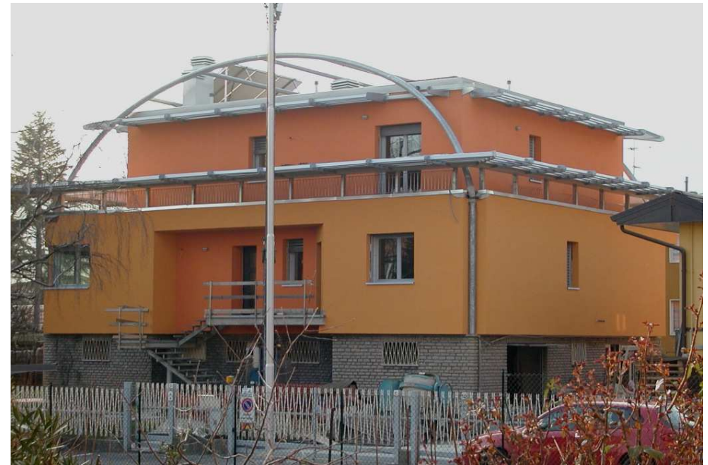
View of the building during renovation.
