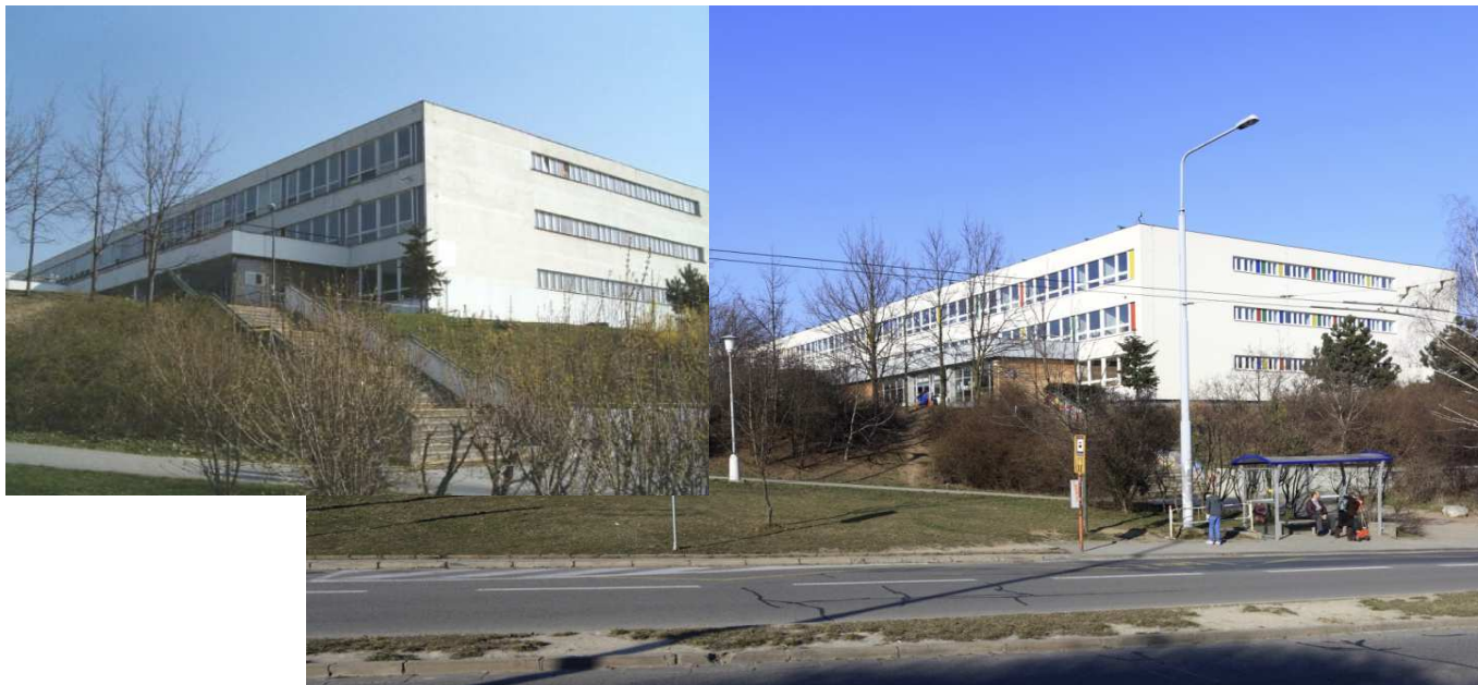
Street view of the school's main block before (left) and after (right) renovation. [1]
