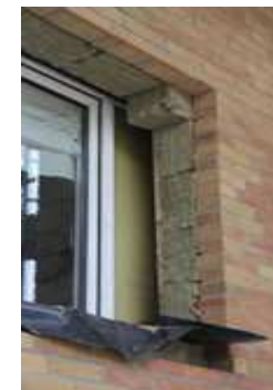
Facades – during works in upper floors
