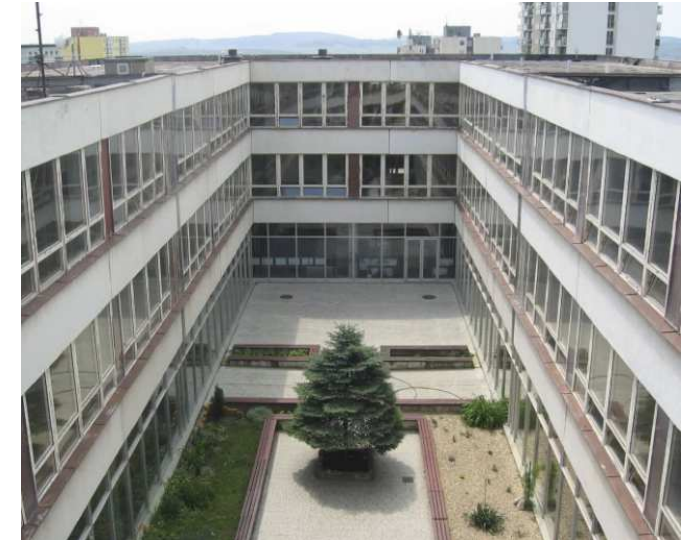
Atrium in the middle of the main block before the renovation. [1]
