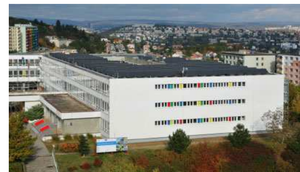
Aerial view of the school's A block with photovoltaic power plant on the roof. [2]
