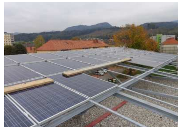
Mounting of the photovoltaic panels on the roof (left picture), pv and solar thermal panels on the south façade (right picture)
