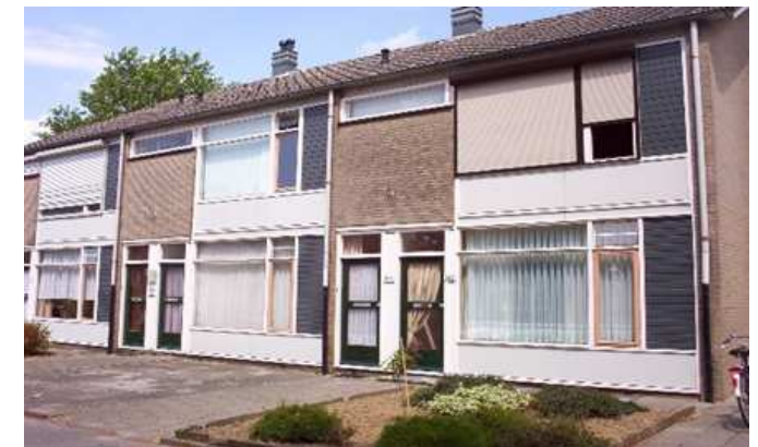
The houses before renovation
