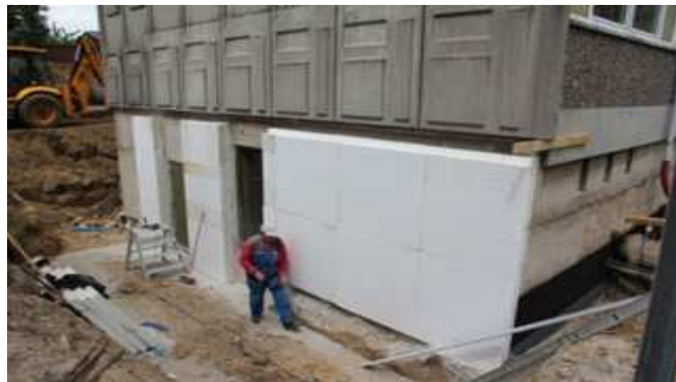
Facades – during works in base floor
