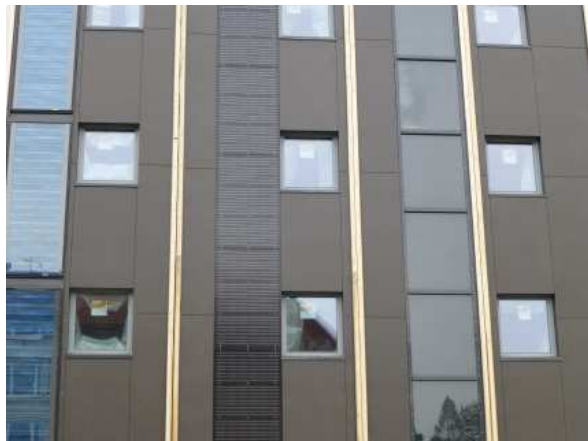
Prefabricated façade elements with integrated active energy production (photovoltaic and solar thermal panels)
