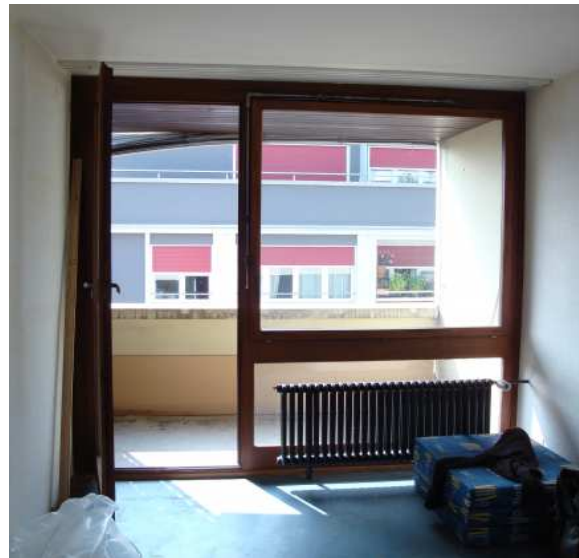
Living room before renovation
