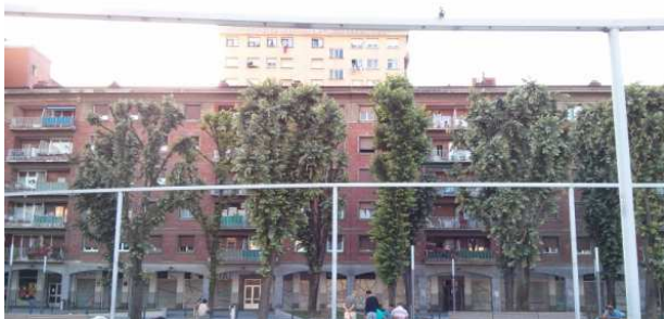
Building before renovation
