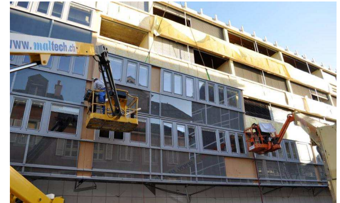
New prefabricated modules during the renovation
