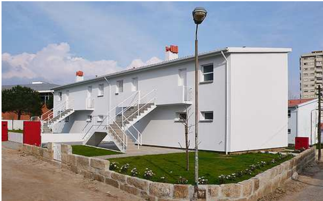
Back facade of the renovated buildings
