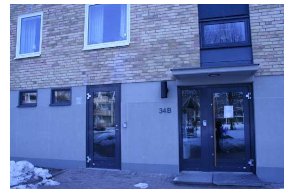
New windows and entrance
