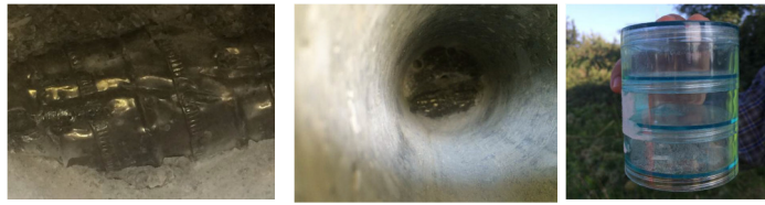
Fig.2. Tendon Inspection and Grouting Sampling (CI)
