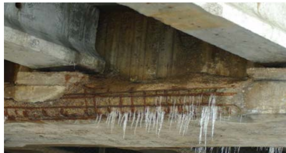
Freeze-thaw damage
