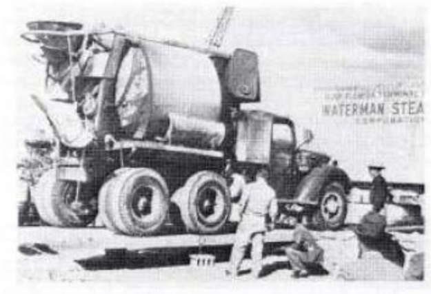
Test of prestressed slab, USA, 1954
