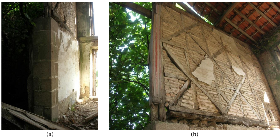
Figure 7-4 Loading on the tested masonry wall: (a) second level granite masonry wall; and (b) third level timber and brick infill masonry wall
