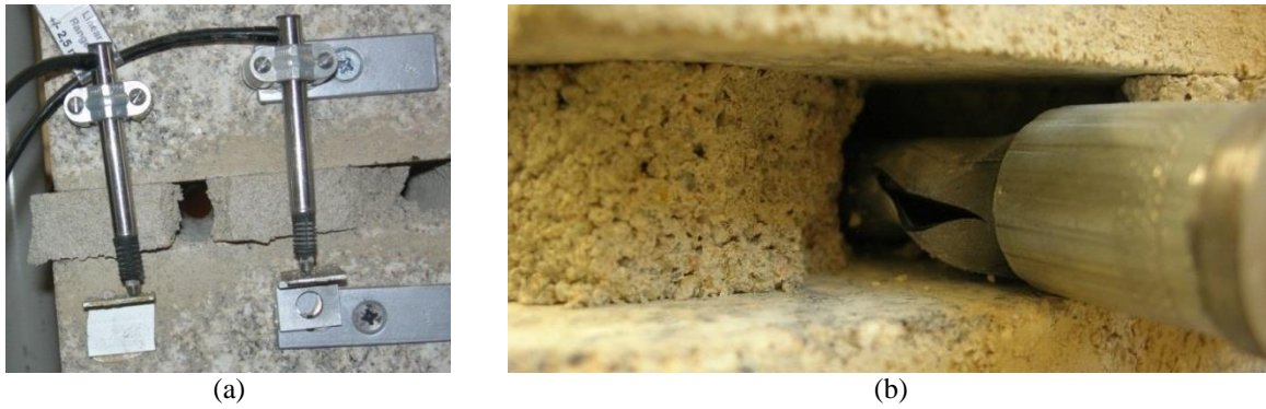
Figure 3-8 Second trial issues: (a) mortar breaking out on the back of the specimen; and (b) lack of confinement of the tube-jack leading to rupture
