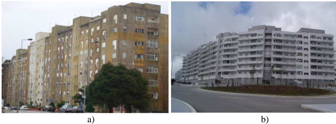
Figure 1 Buildings general aspect. a) Before the intervention, b) After
