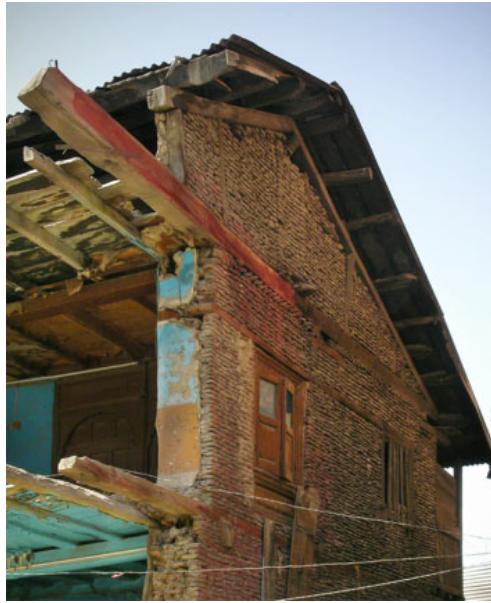
Figure 21: Taq timber - laced system, Srinagar, Kashmir, India (credits: R. Langenbach).
