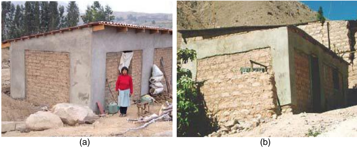
Figure 25: Reinforced model after seismic test reinforced house after the 2001 earthquake Adobe buildings with external wire mesh reinforcement ( Blondet & Aguilar, 2007 )
