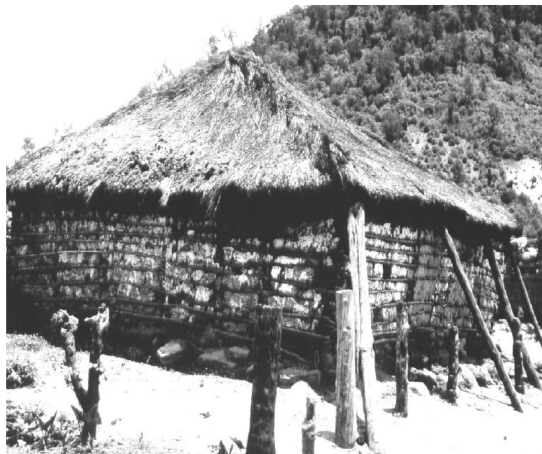
Figure 11: Wattle-and-daub structure that survived after a heavy earthquake in Guatemala (Minke, 2001)
