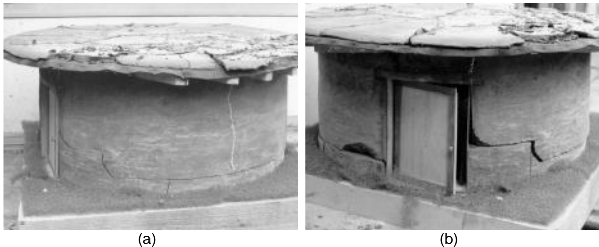
Figure 15: Circular RE models (a) first crack appeared only after 3 rd stroke and (b) after 6 th stroke a small part was separated ( Minke, 2001 )
