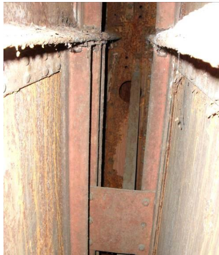
Figure 21 – Side views of the interior of the walls.
