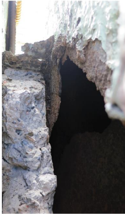
Figure 31 – Concrete applied on the pinnacle valleys.
