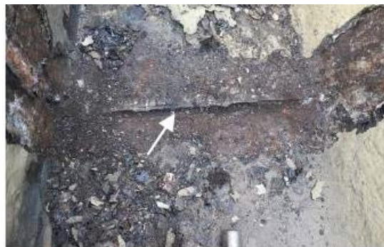
Figure 30 – Gutter being mechanically cleaned.
