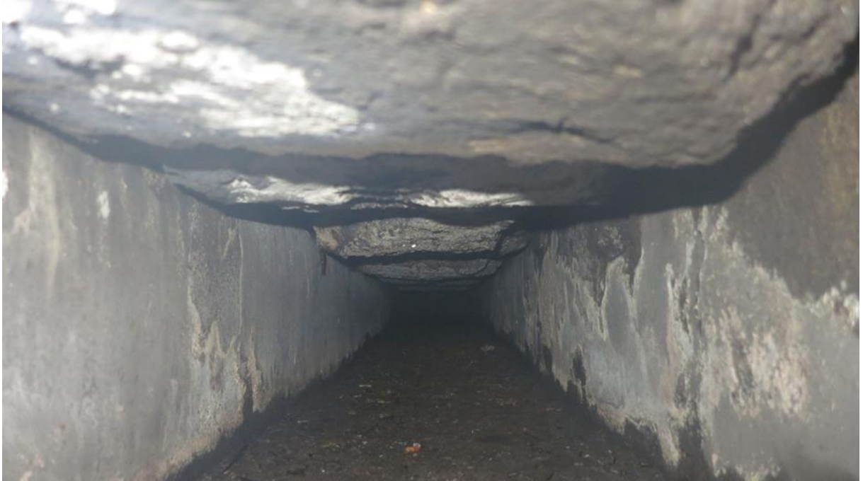
Figure 23 – Crawl space beneath the floor.
