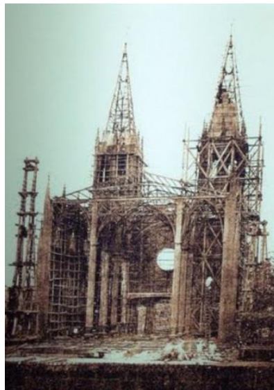
Figure 6 – Construction of the Steel Church (Conservation and Development Foundation 2014).
