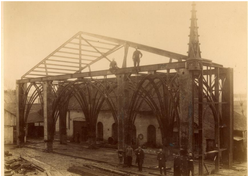
Figure 5 – Assembly of a part of the basilica in a factory (Conservation and Development Foundation 2014).
