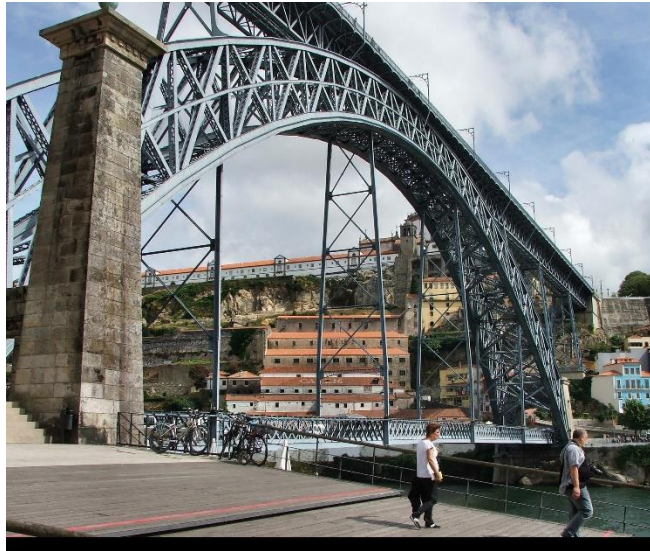
Figure 28 – Luis I bridge, in Porto, Portugal.
