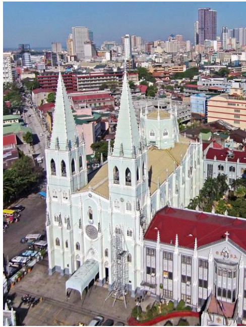
Figure 8 – General view of the Church.
