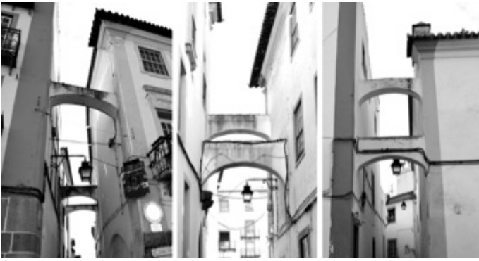
Figure 6. Different reinforcing counter-arches in the historical centre of Évora (credits: CI-ESG).
