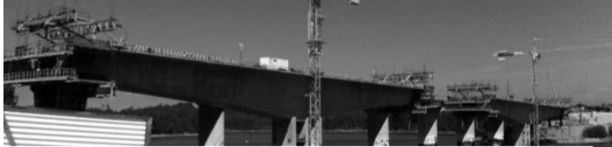
Segmental Prestressed RC Bridge
