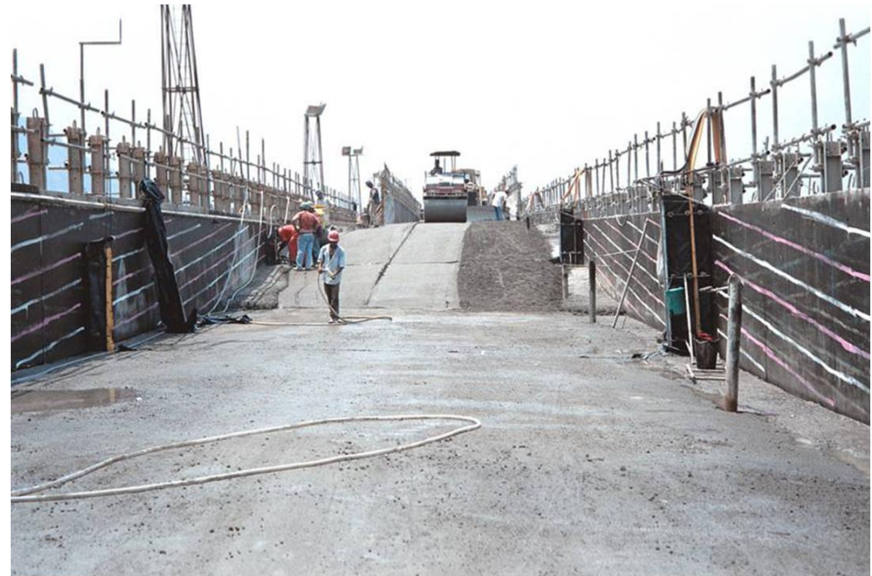
Sloped lift layer (0,3m) of RCC placement at Lajeado HPP (Brazil).
