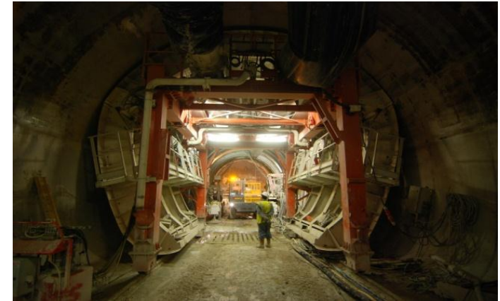
Tunnel lining formwork
