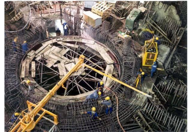
Itaipu powerhouse – 2 nd stage construction (2003)
