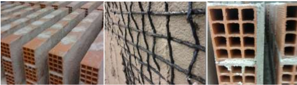
Fig. 18 - Construction of the walls and application of reinforcement mesh
