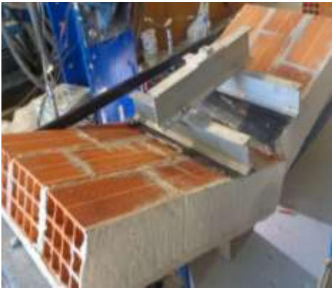
Fig. 22 - Typical failure mode in unreinforced specimens
