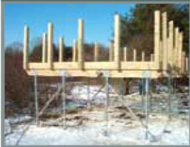
Braced brackets and placed tension anchors for support
