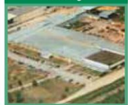
MacLean-Dixie HFS™ manufacturing facility
