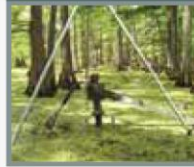
Helical steel piles being installed into swampland
