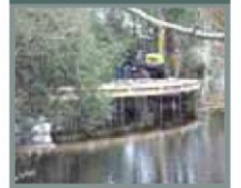
Concrete pile caps cast to support timber columns
