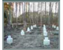
Concrete pile caps cast to support timber columns
