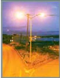
Up and running with minimal manpower and equipment
