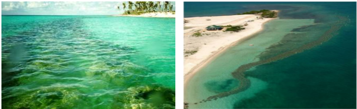
Figure 2.4: Examples of submerged breakwaters.
