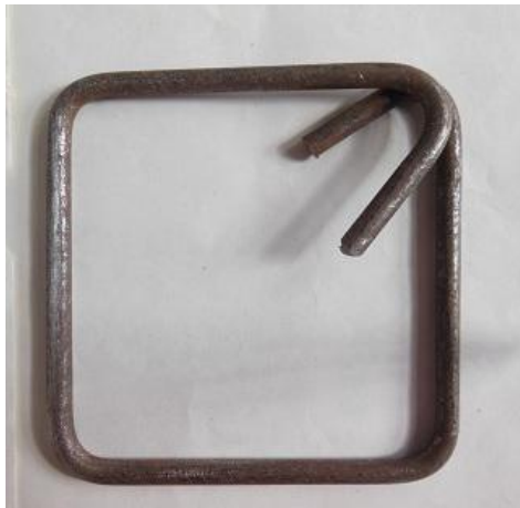
Figure 6 Conventional stirrups
