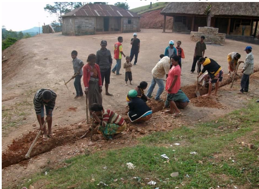
Picture 5 – The community digging the water pipe ditch
