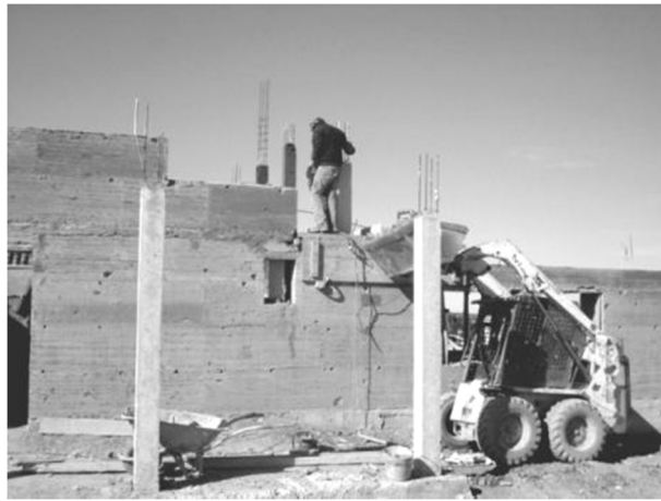
Figure 2.5 – Construction of a new rammed earth house in Colos (Odemira), Portugal.
