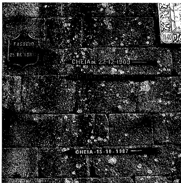
Fig. 3. On the tower of the "Passeio 25 de Abril" Place, benchmarks of floodwaters indicating the occurrence of various floods (AD 1909, 1959, and 1987) in the city of Ponte de Lima (from Martins, 2009). Water heights have been measured with a laser distance metre.
