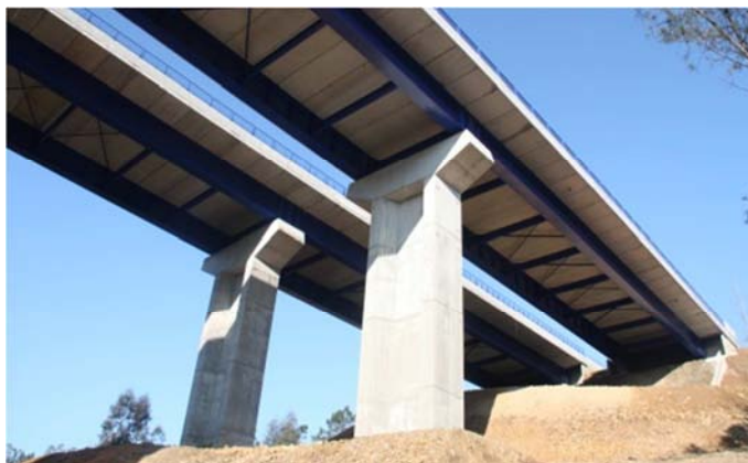
Figure 7.10. Sousa River Bridge, inferior side view (provided by Teixeira Duarte, S.A.).
