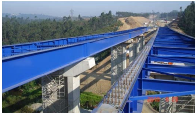
Figure 7.5. Metallic girders, overview (provided by Teixeira Duarte, S.A.).
