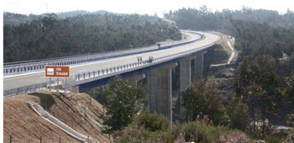
Figure 7.1. Sousa river bridge, overview [99].
