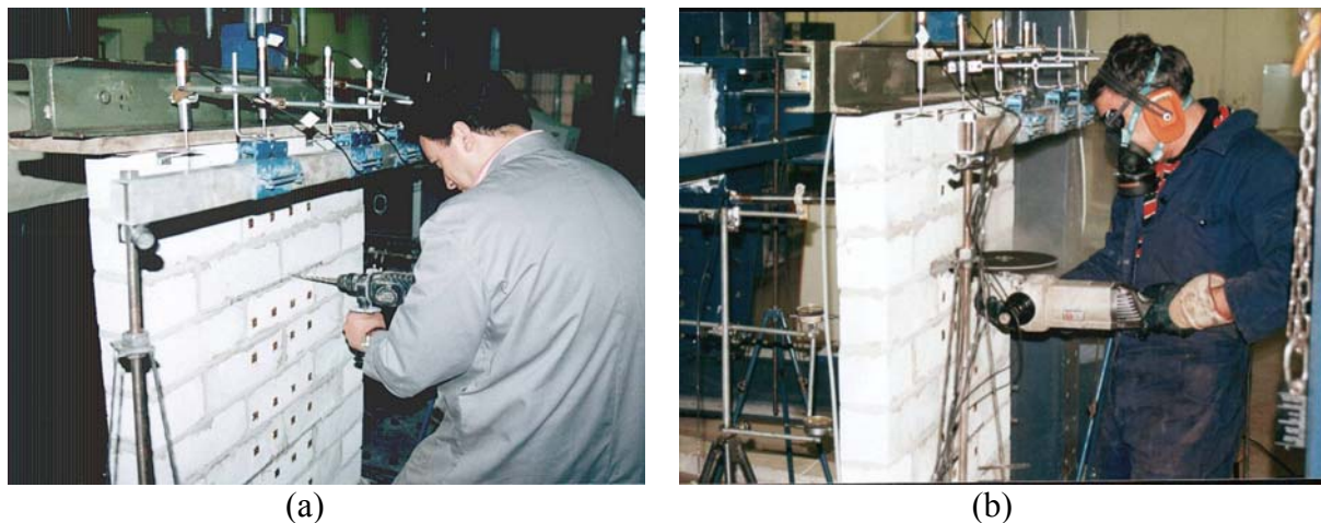
Figure 12 - Mortar removal: a) by stitch drilling b) saw cutting.
