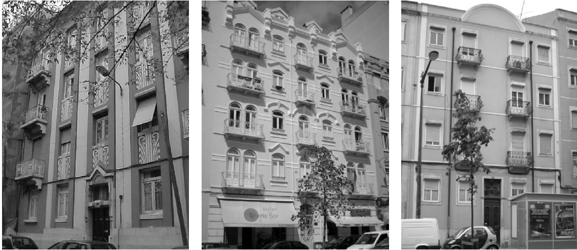
Figure 1.13 – Examples of “gaioleiro” buildings, Lisbon, Portugal.
