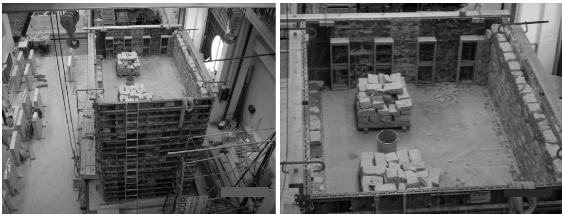
Figure 2.4 – Construction of the non-strengthened mock-up.
