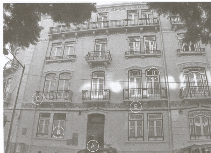
Figure 1.14 – Facade of a “gaioleiro” buildings (Appleton 2005).
