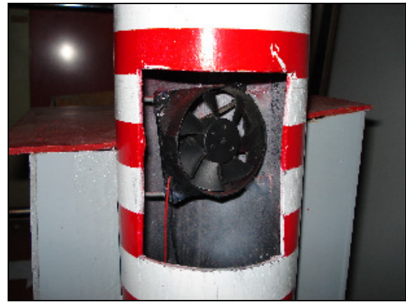
Figure 6. Fan inside the chimney
