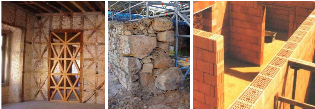
Figure 1: Examples of different masonry types (from left to right): timber braced “Pombalino” system emerging after the 1755 earthquake in Lisbon; irregular stone wall with a complex transverse cross section (18 th century, Northern Portugal); typical European unreinforced masonry used in areas of low seismicity using thick blocks to comply with thermal and sound regulations.
