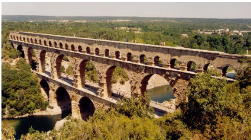
Figure 2.7 – The long aqueduct Pont du Gard, Nîmes, France.
