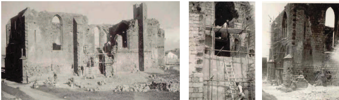
Figure 11. Historical photographs (1940, 1941), showing conservation works and the deficient condition of the church
