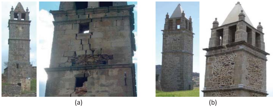
Figure 9 Mogadouro Clock Tower and conservation works: (a) before; (b) after.
