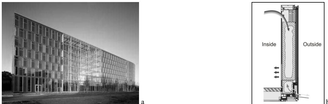
Figure 1. Capricorn Haus Façade, Düsseldorf (a) and section façade detail (b). Reference: FSL, 2010.
