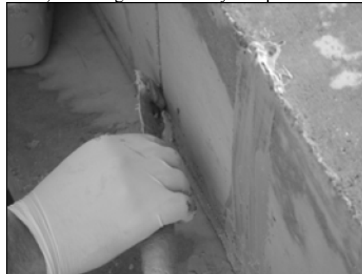
4) Filling up the slits with adhesive
