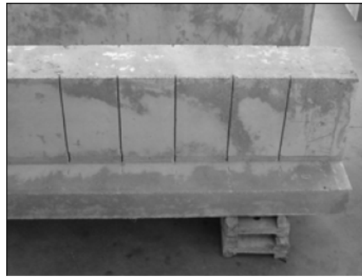
2) Cleaning of the slits by compressed air
