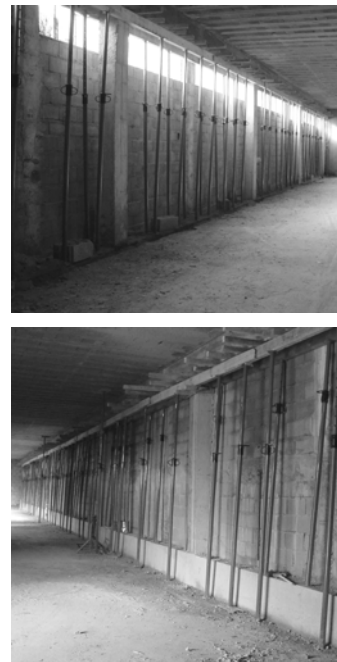
Figure 2 – Frames supporting the slab.
