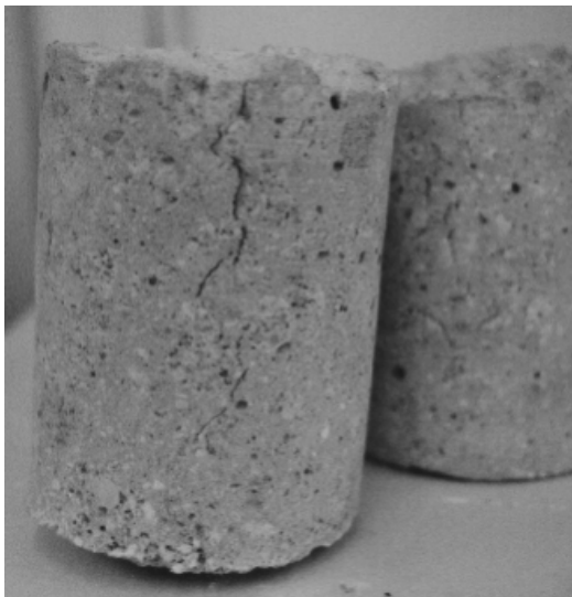
Figure 11 – Some drilled cores had shrinkage cracks.
