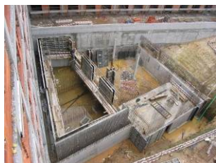
Figure 7. Rainwater tank (construction phase).
