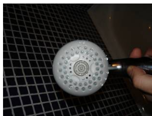
Figure 8. Low flow showers.
