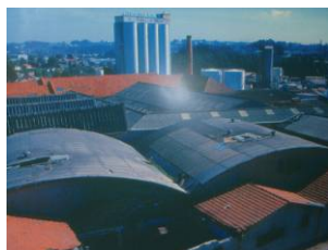
Figure 5. Aspect of the local before the intervention.
