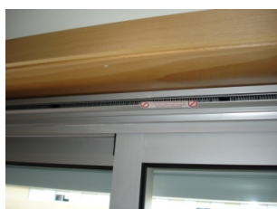
Figure 10. Ventilation grids on window frames.
