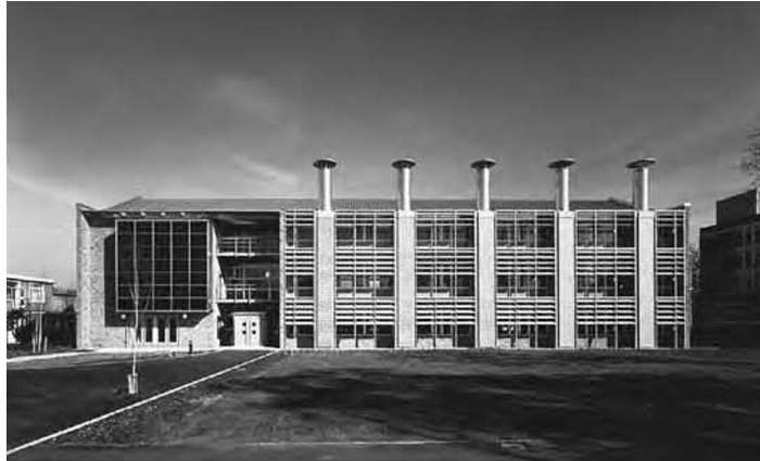
Figure 2.7. Environmental Building (EB), Building Research Establishment (source: Thomas & Stevens, 1996).
