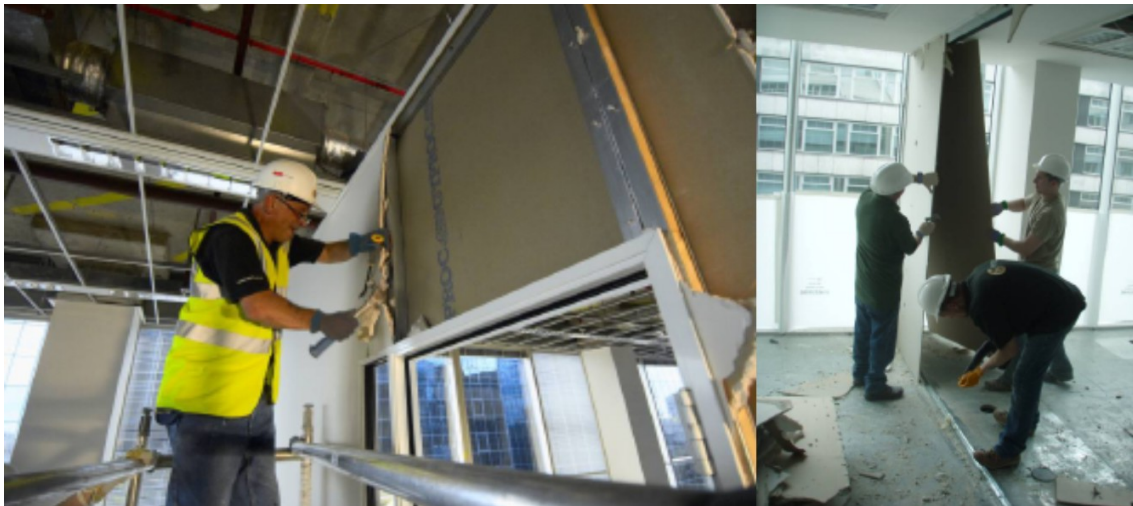
Figure 3.3. Recovery of plasterboard (Lee, 2006).
