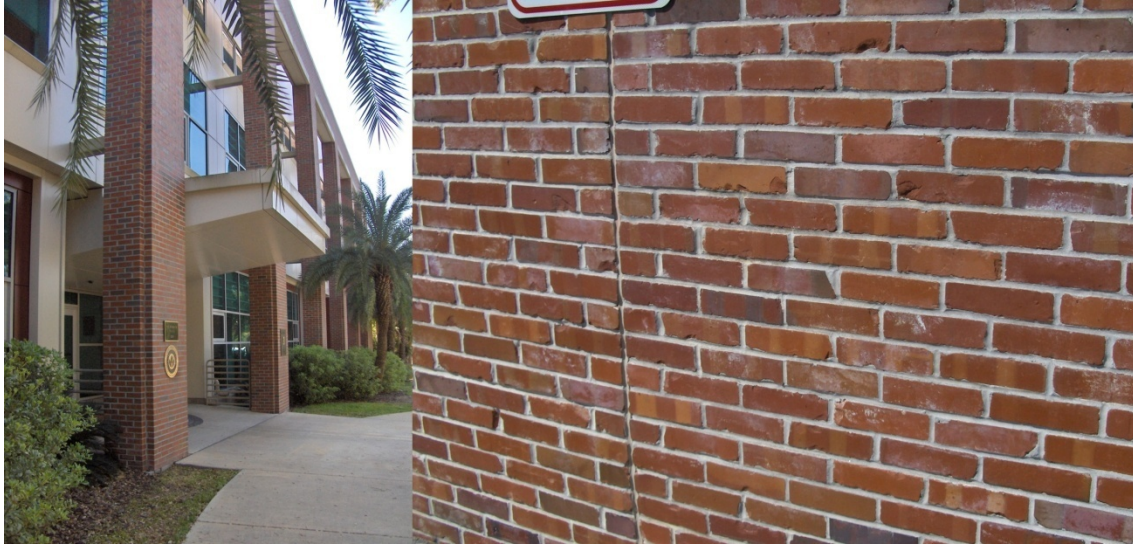
Figure 3.2. Rinker School of Building Construction, University of Florida: bricks from demolished building were reused in the new building.
